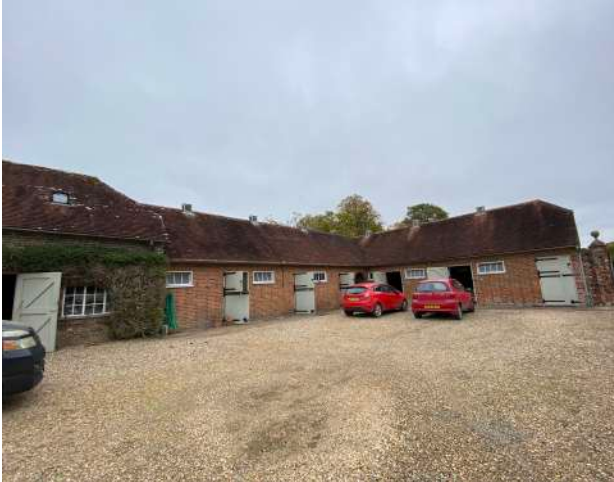
Image 1: Southern elevation of the building
