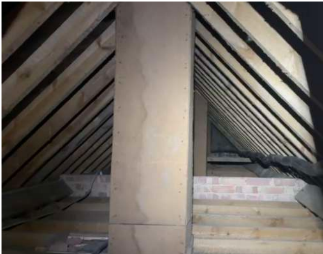
Image 9: Void B - only viewed through a small panel
