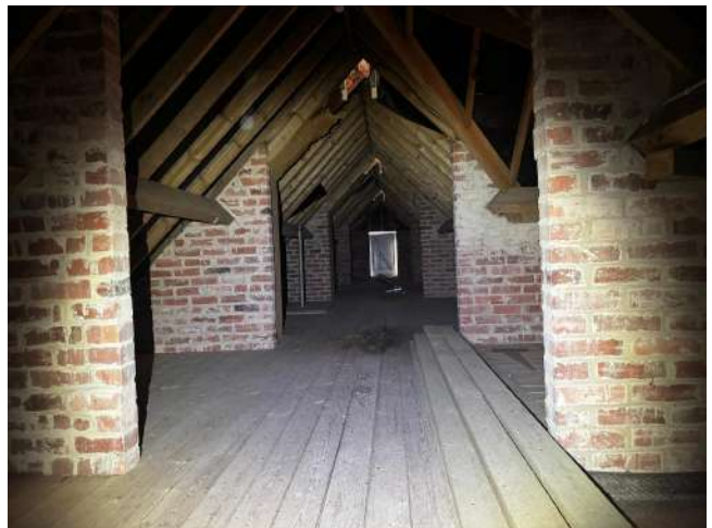
Image 4: Void A, looking towards hayloft door at southern end
