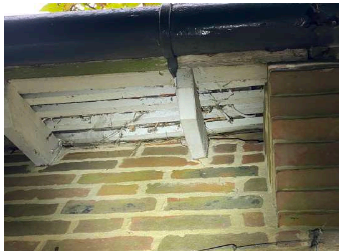
Image 12: Eaves access at the northeastern corner
