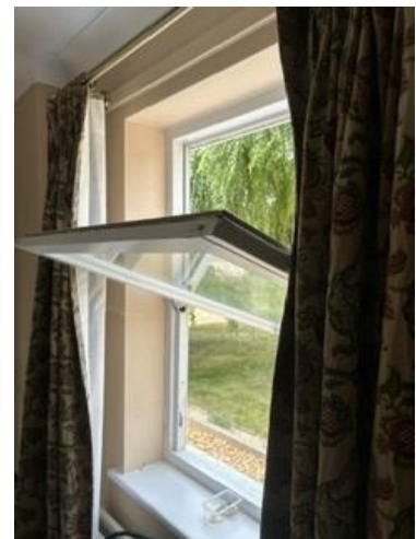
Existing window to first floor of two-storey modern wing
