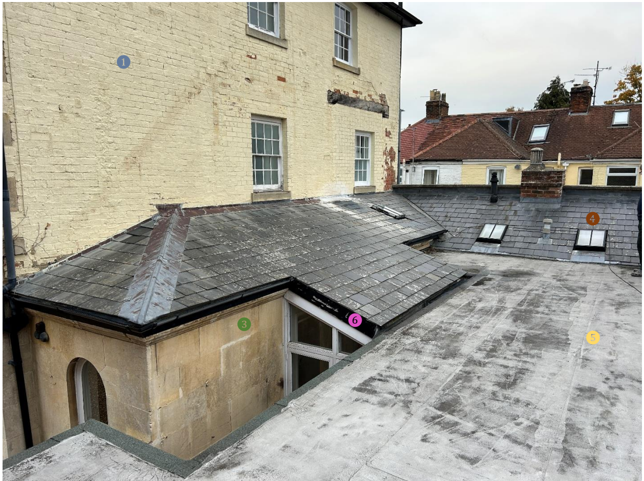
View from top of flat roof looking north.
