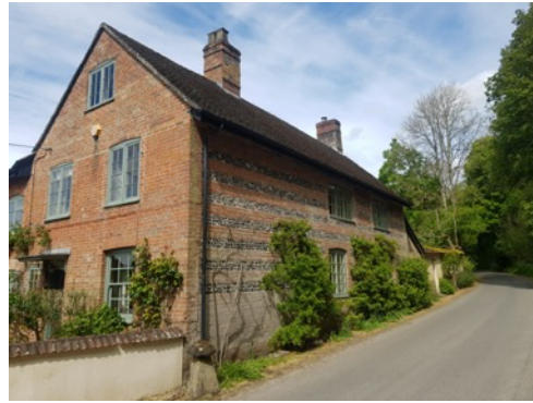
Photo 2: B1 - East facing elevation
