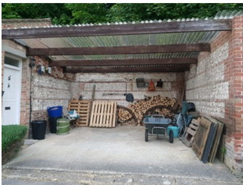
Photo 9: B2- - internal view of carport
