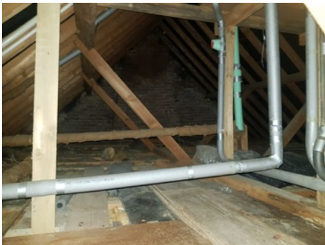
Photo 5: B1 - Internal view of loft element
