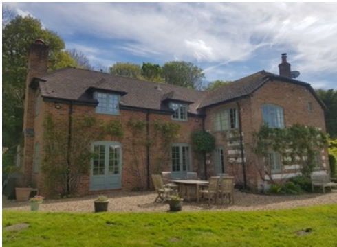
Photo 3: View of the residential dwelling (B1) from the west
