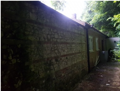
Photo 7: B2- Rear east-facing elevation
