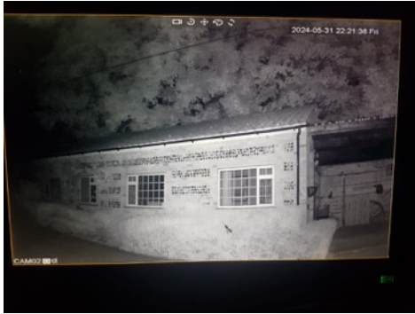
Photo 13: B2 – infrared camera view
