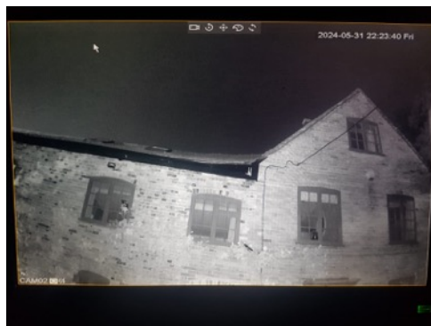
Photo 12: B1 – infrared camera view
