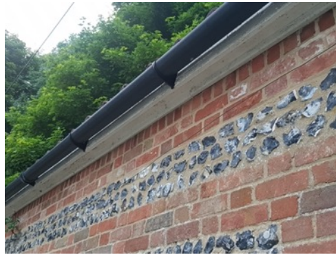
Photo 8: B2 - Soffit without damage.
