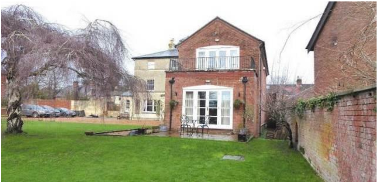
Fig: Melbourne House from the southeast
