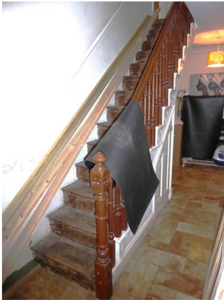
Fig 4.10: Main stairs to first floor
