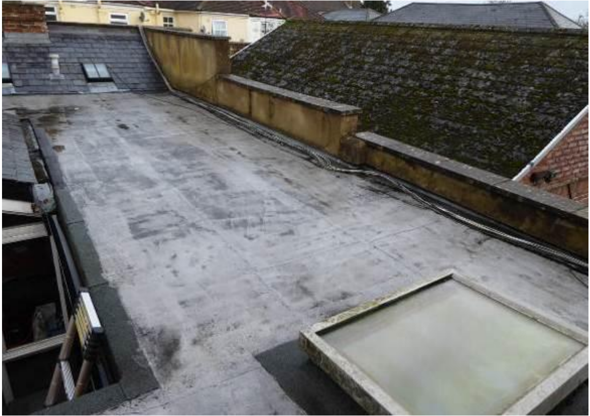
Fig 3.14: East side flat roof over existing kitchen
