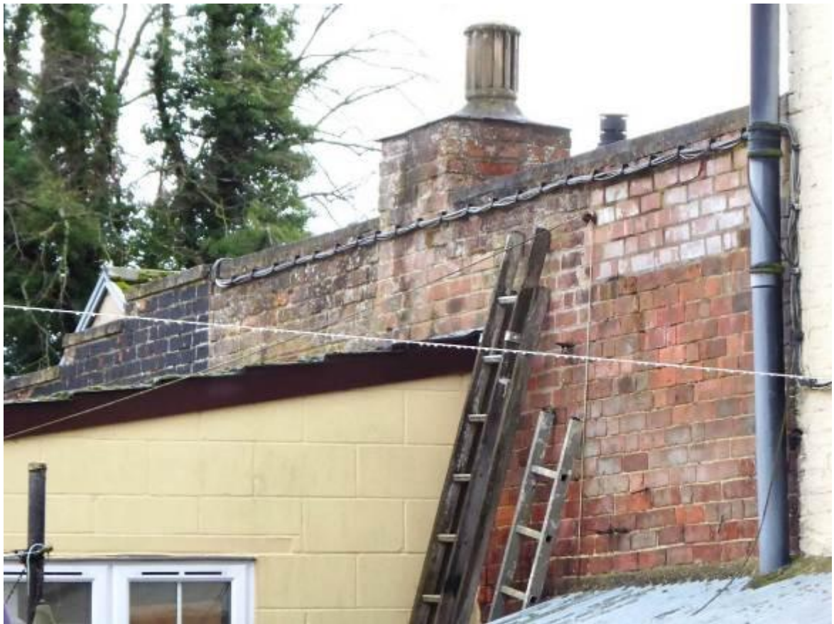
Fig 3.4.10: Rear (north) wall to kitchen
