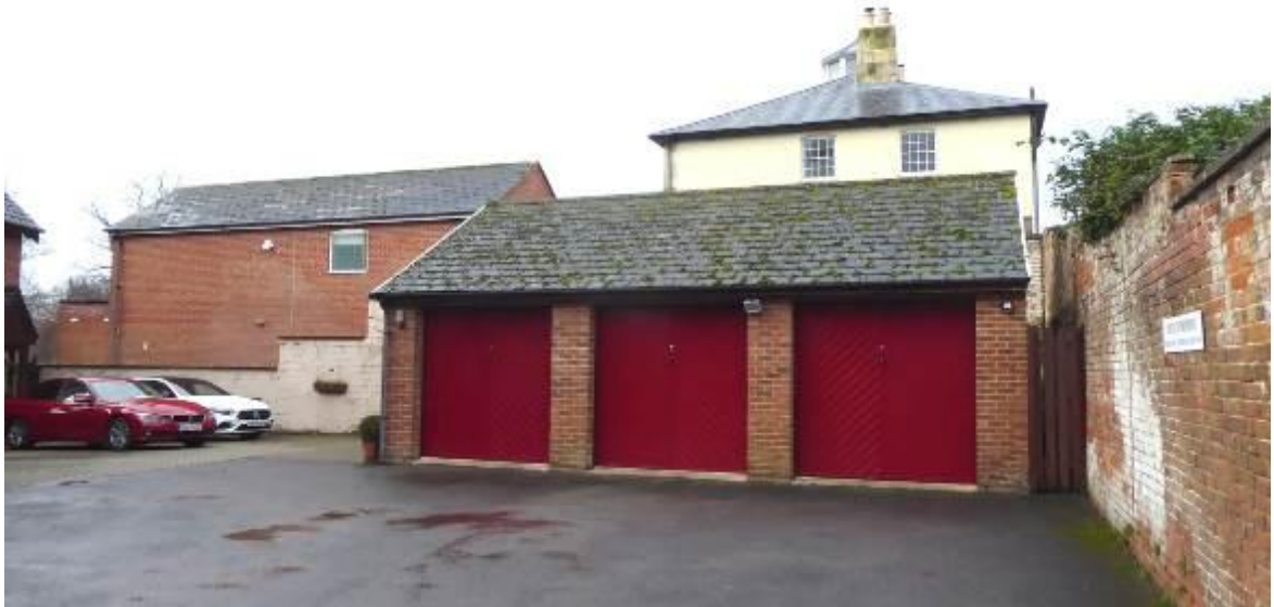
Fig 2.1.4: Melbourne House from Melbourne Mews
