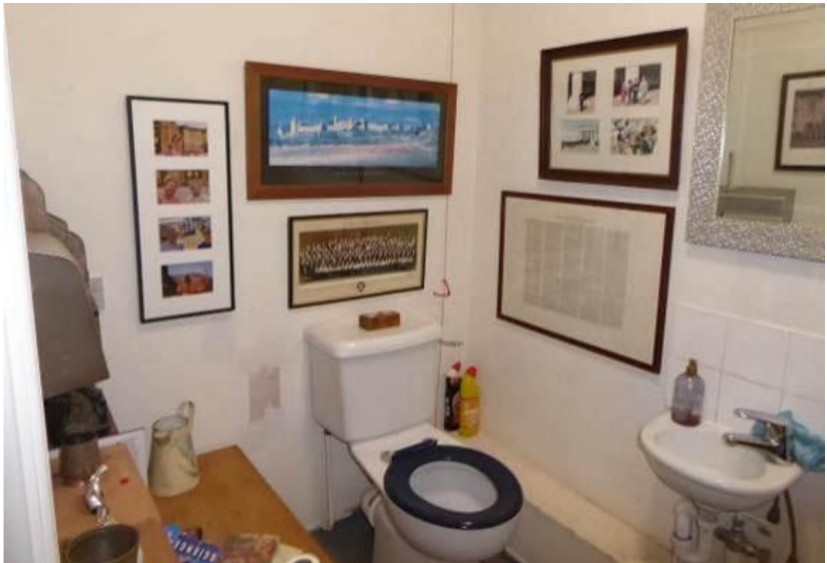
Fig 4.6: Ground floor cloakroom
