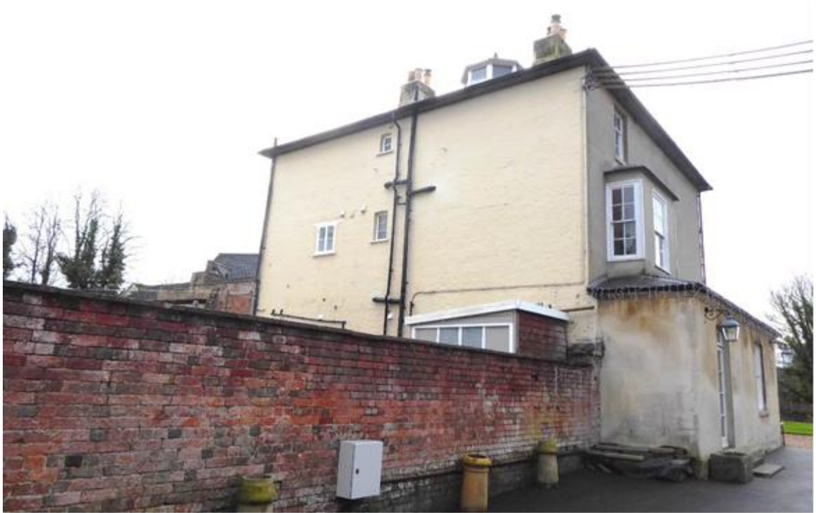
Fig: 2.2.1: Melbourne House from the northwest
