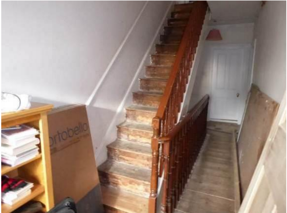
Fig 4.17: Stairs from first to second floor
