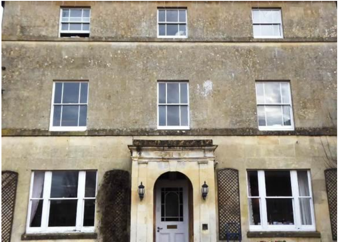
Fig 3.5.2: South elevation windows
