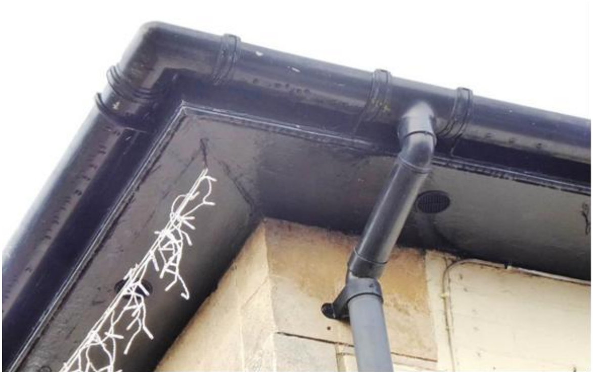
Fig 3.3: Eaves to main house
