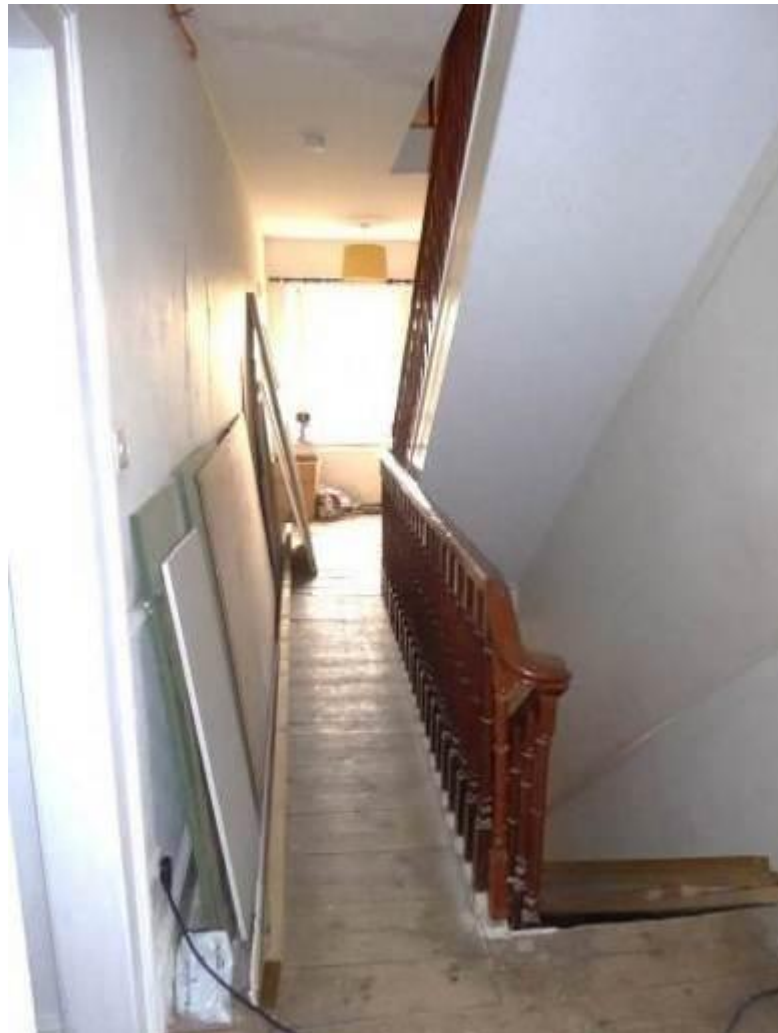
Fig 4.11: First floor landing
