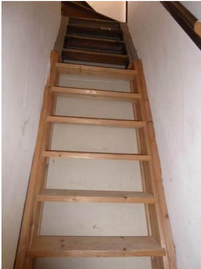
Fig 4.23: Stairs to cupola
