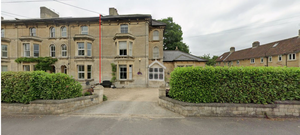
Figure 1 - Existing Street Scene, 107 Trowbridge road with Party wall marked in red
