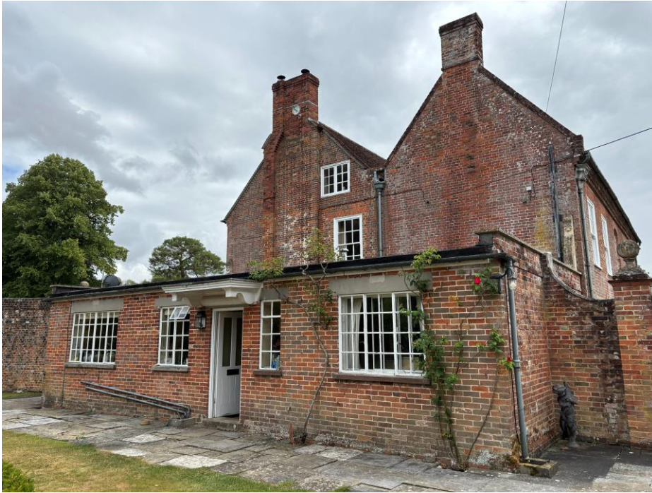
Fig.6 Single-storey flat-roofed kitchen extension on the northern end of the house – note the Crittal windows with concrete lintels and cills
