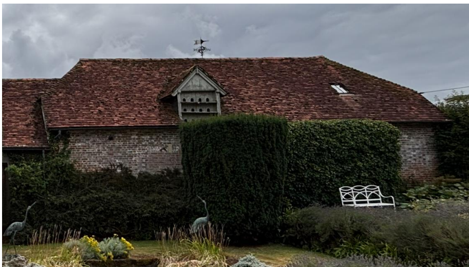
Fig.13 Rear of the garage element of the building with timber dove-cote at eaves level as seen from the sunken garden to the south of the house
