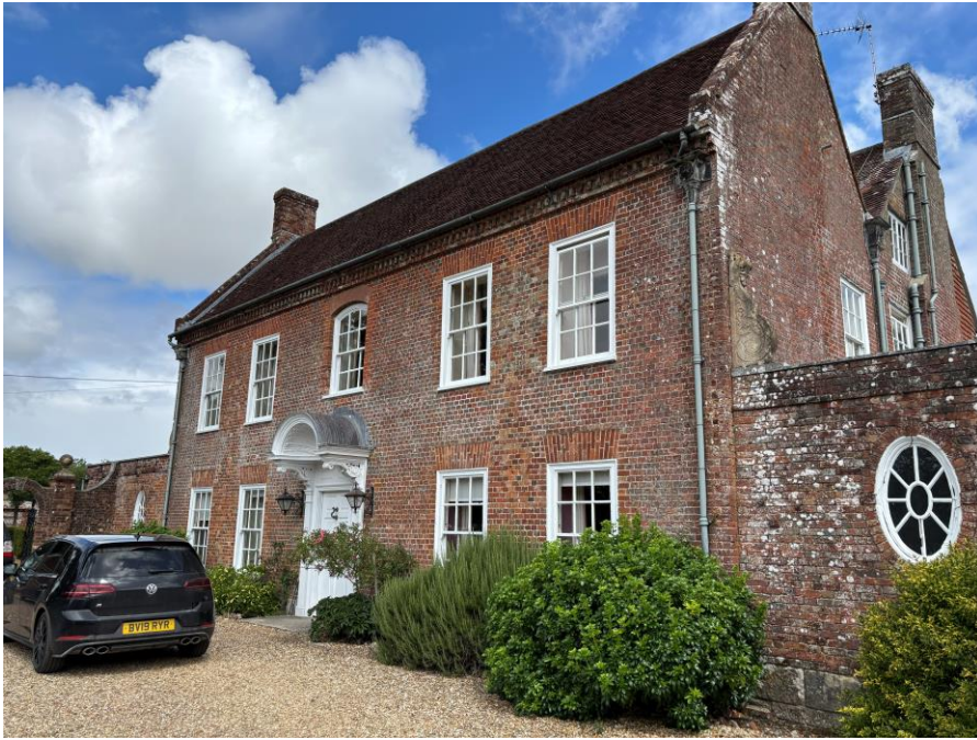
Fig.4 West front of the house – existing extension set behind the wall to the left
