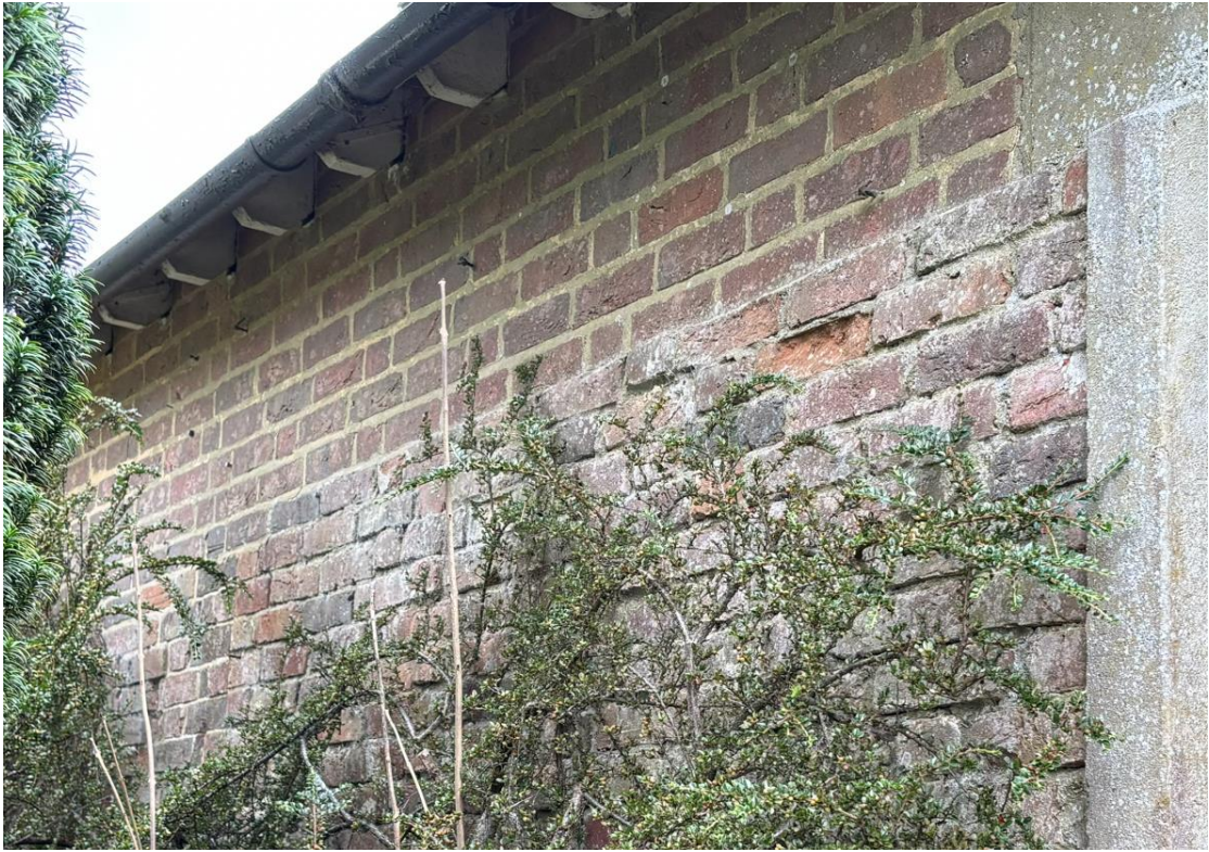
Fig.19 Closer view of the older brickwork with modern above
