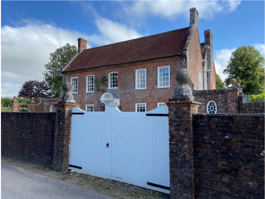
Fig.3 View of the house from the road with tall brick boundary walls in front – existing single-storey extension screened from view
