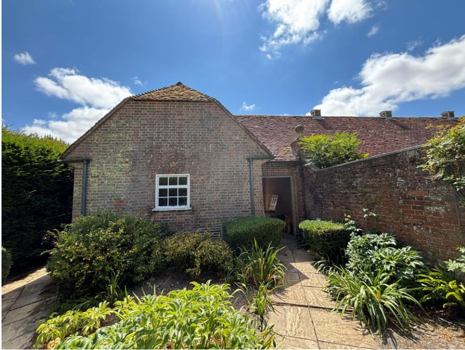
Fig.17 North side of the stables range with throughway
