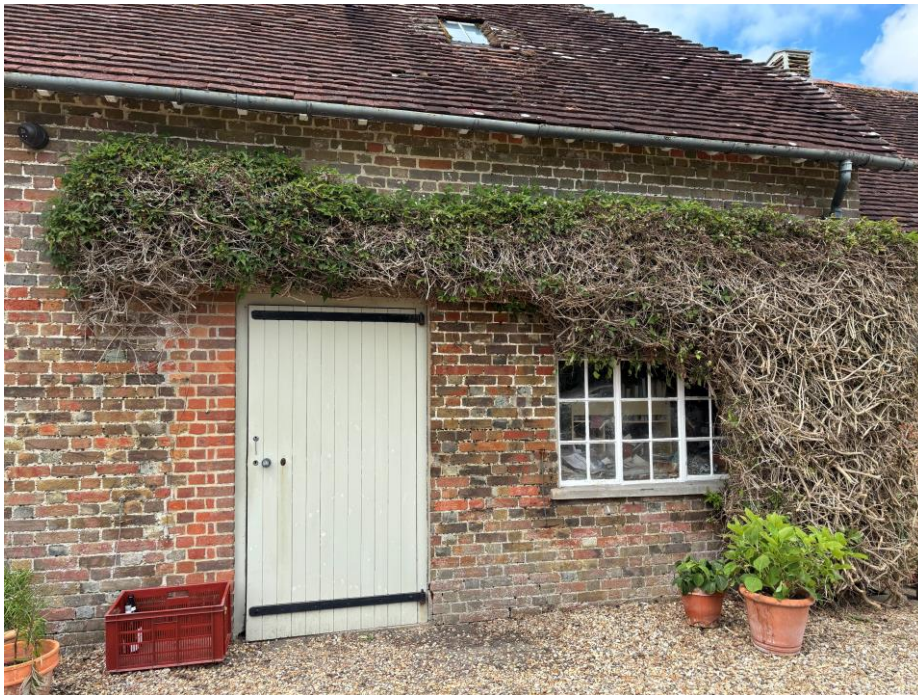
Fig.12 Personnel door and window at the eastern end of the garage range (note the variation in the brickwork to the left of the doorway where it might have been wider)
