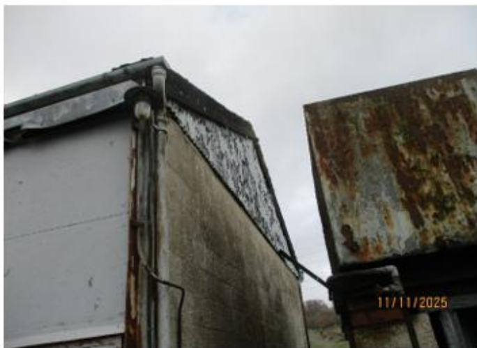
Photo 13: Gable end of 'B1'.
