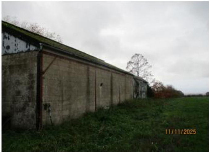
Photo 10: Rear elevations of 'B1 and B2'.
