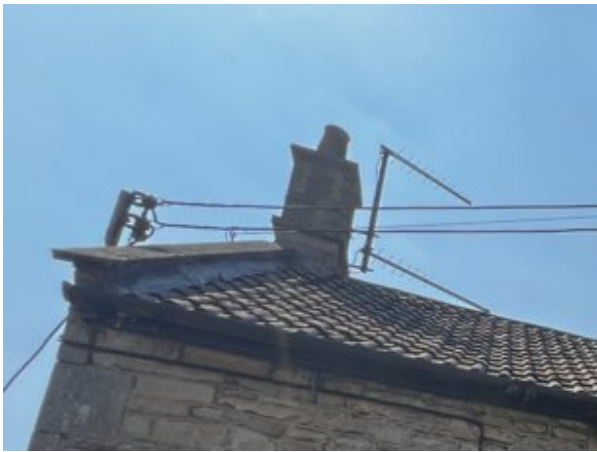
Photo 11: Gap Under Lead Flashing at Eastern Gable End of Cottage
