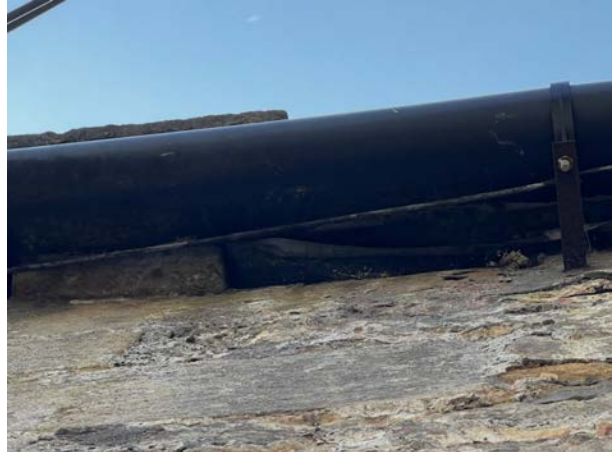
Photo 10: Gap Under Lead Flashing Western Chimney of Cottage
