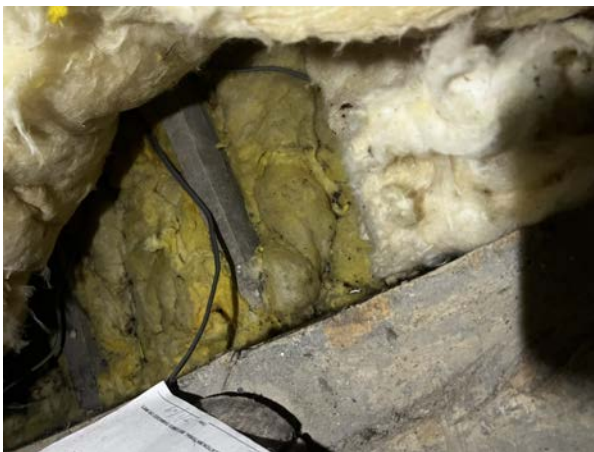
Photo 17: Mice Droppings On and Under Insulation
