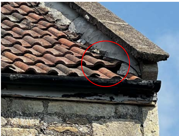
Photo 11: Gap Under Lead Flashing at Eastern Gable End of Cottage
