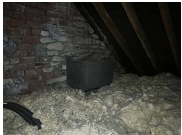
Photo 18: Disused Void Water Tank
