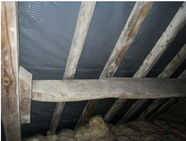
Photo 17: Mice Droppings On and Under Insulation
