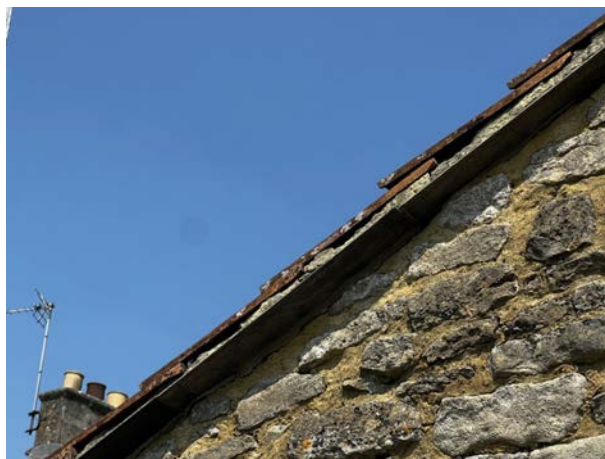
Photo 26: Garage Southern Gable End Tiles
