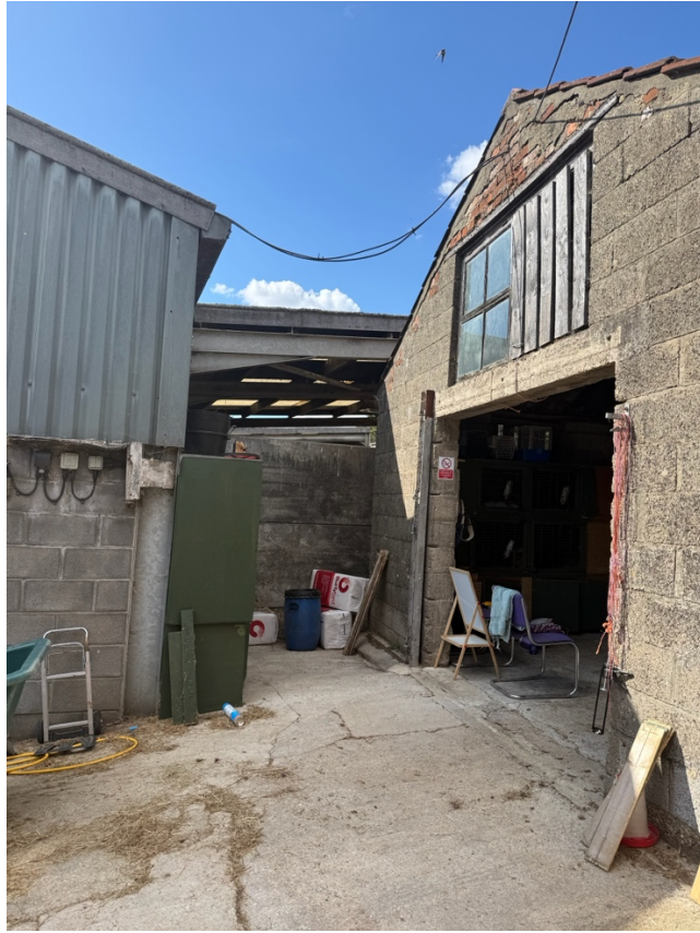
Figure 5 – Rear of washroom & store
