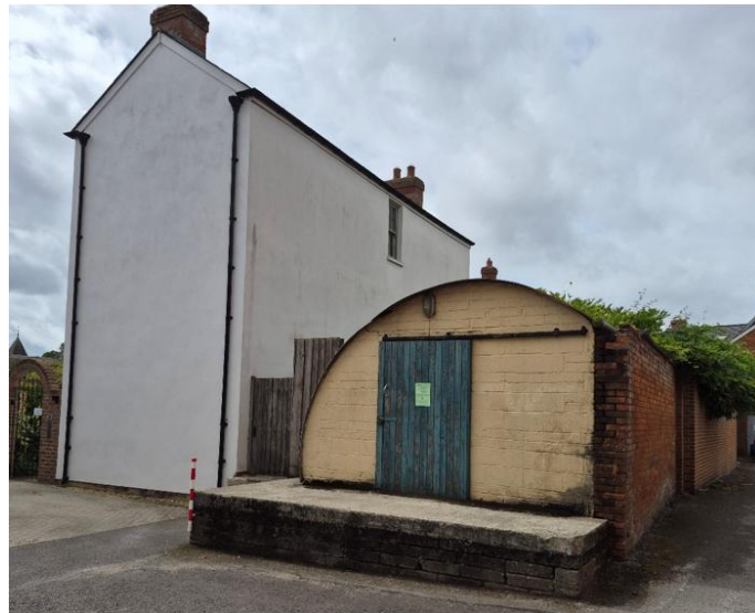
Eastern Elevation with Existing Nissan Hut
