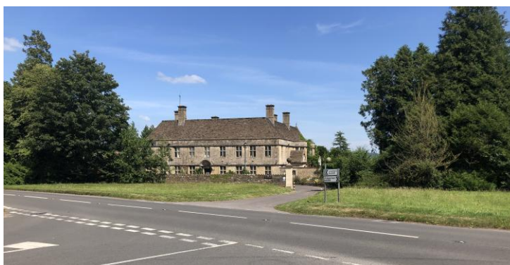
Image 8: Kin House and entrance from Swindon Road
