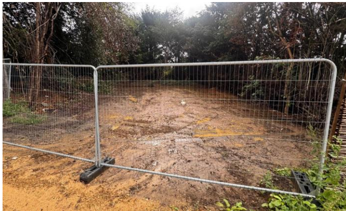
Image 7: The location of the storage building
