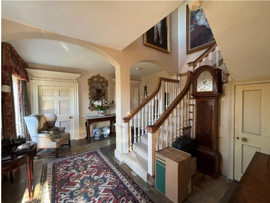
Fig.10 Entrance hall – stair with ramped handrail and turned balusters, and 6-panel doors with moulded architraves
