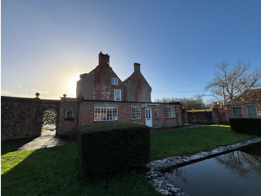
Fig.8 View of the northern end of the house and extension from the north garden
