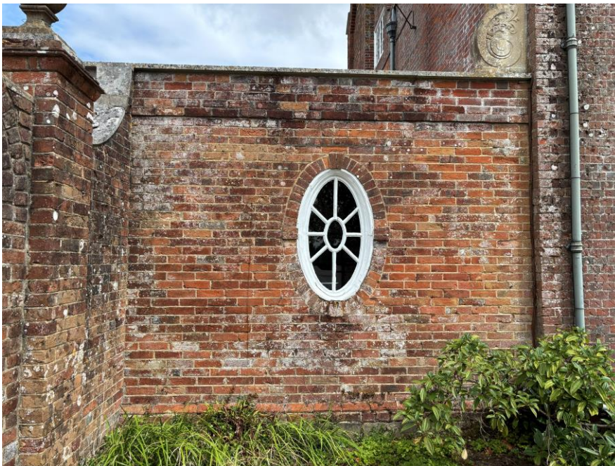
Fig.7 Attractive oeil-de-boeuf window in the west wall of the extension; enclosing wall to the north garden on the left
