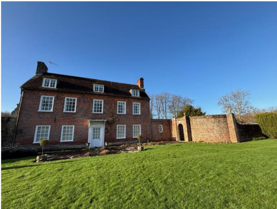
Fig.5 East façade of the house
