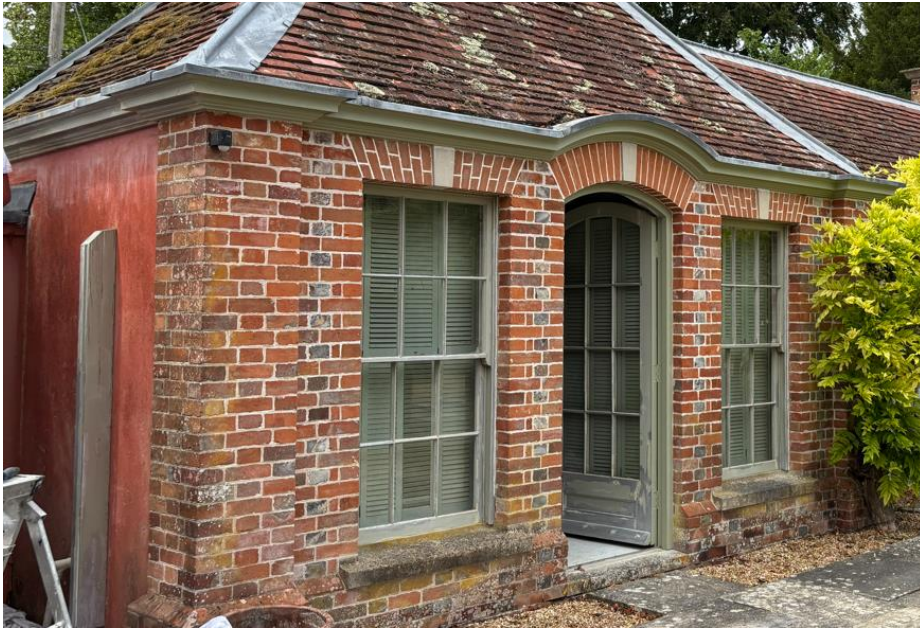
Fig.17 Summerhouse – door and windows with gauged brick arches and keystones
