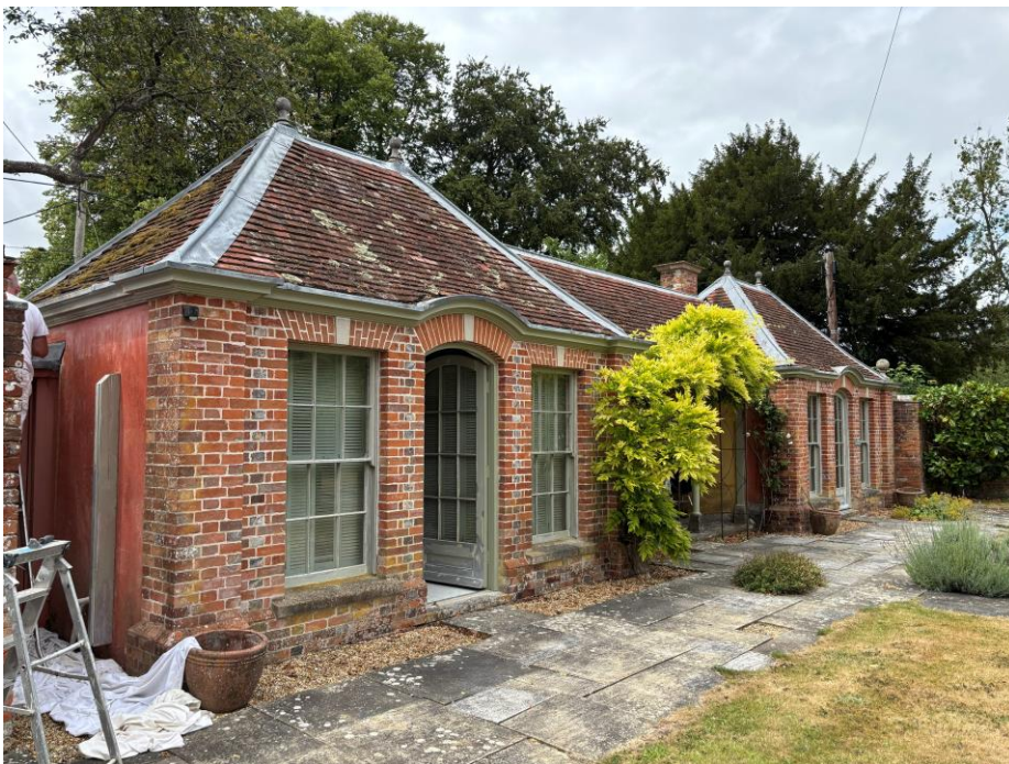
Fig.9 Recently constructed summerhouse to the north-west of the extension
