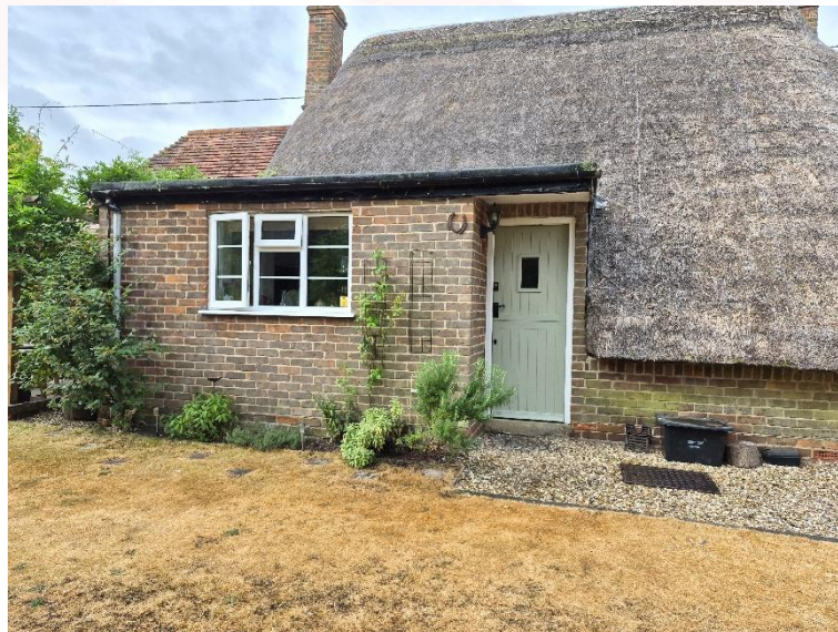
Figure 1: North eastern elevation of property
