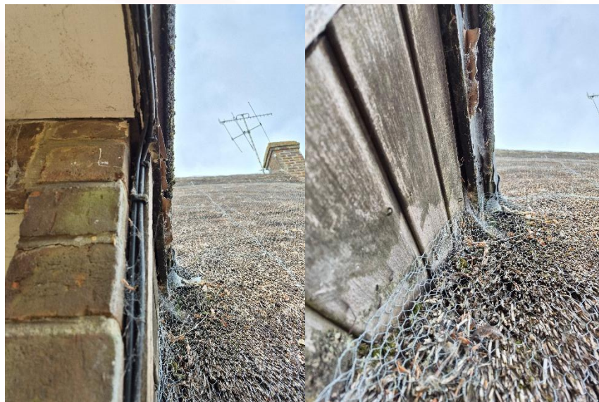
Figure 4 and 5: Timber cladding on the northern elevation
