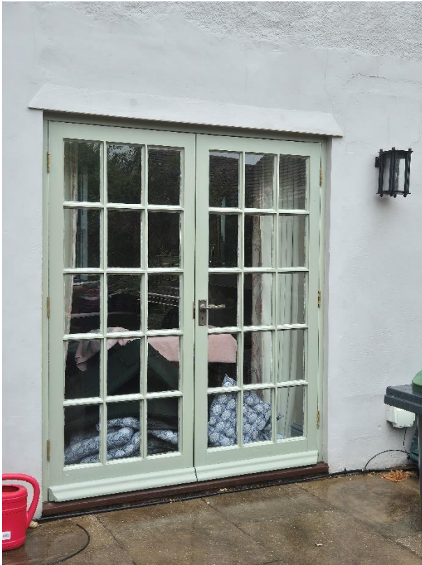
Existing ground floor French doors (bottom right).
