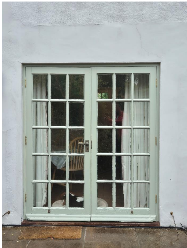
Existing ground floor French doors (bottom centre).
