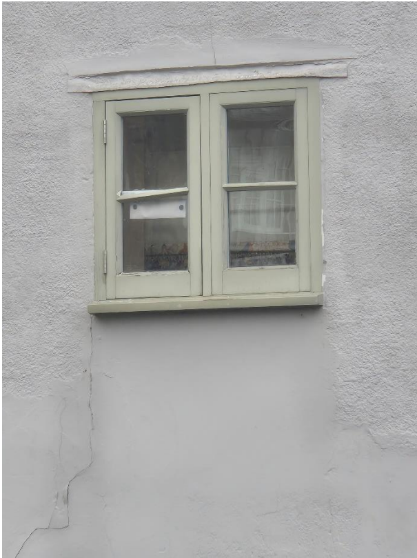
Existing first floor casement window (middle centre).
