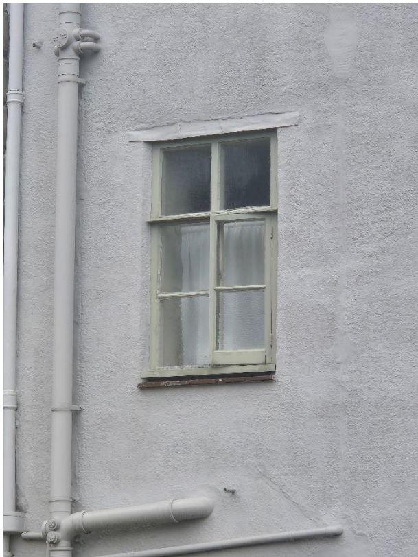
Existing first floor casement window (middle left).
