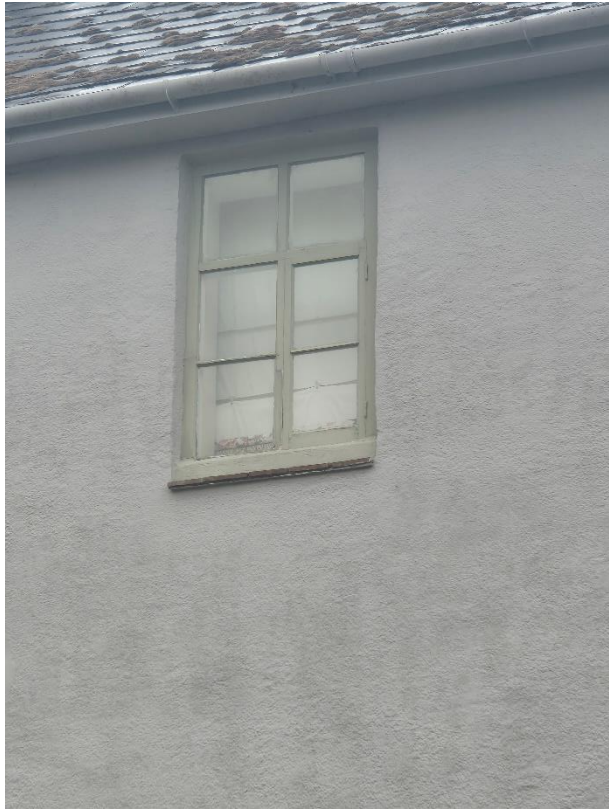
Existing second floor casement window (top centre).
