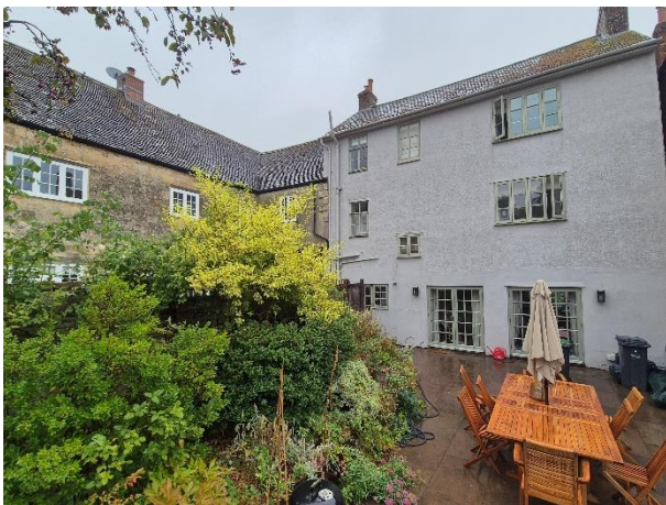
Rear elevation showing existing fenestration.
