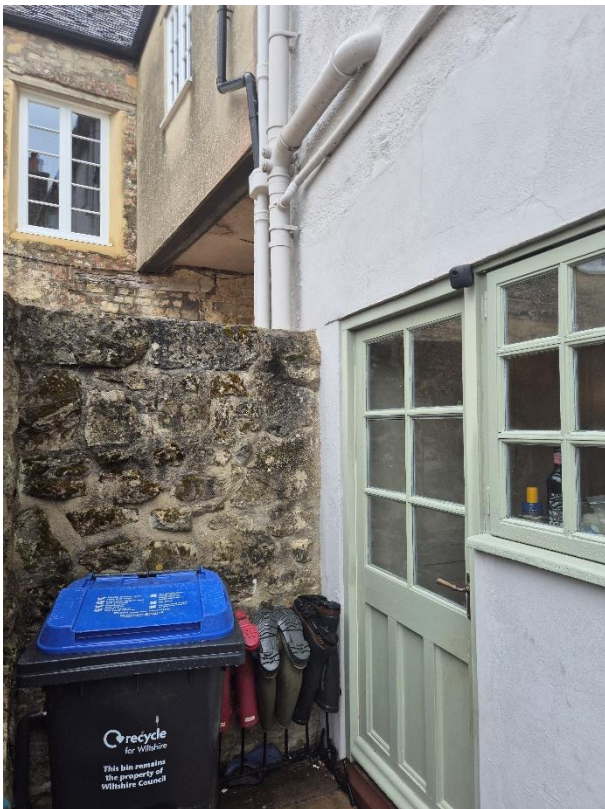
Existing ground floor single door & sidelight (bottom left).
