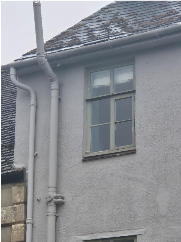
Existing second floor casement window (top left).
