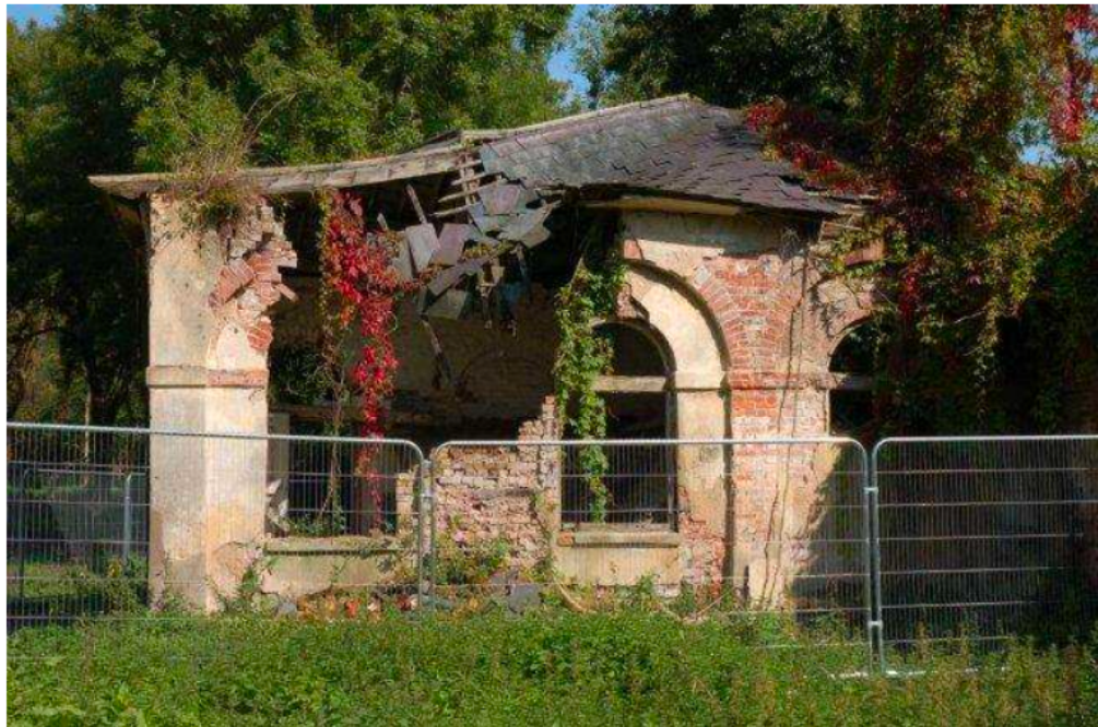
South elevation of south wing - 2015
