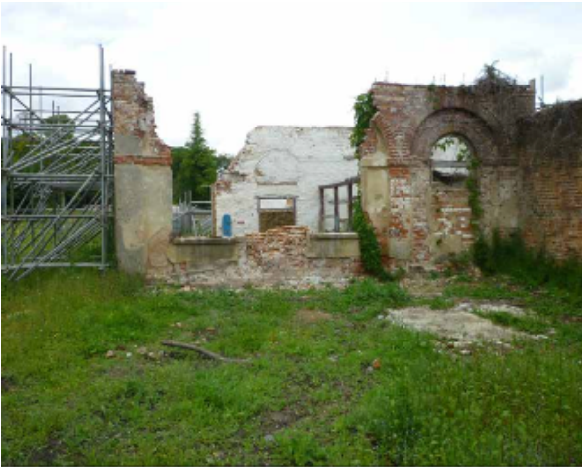
Figure 1: South elevation of the south wing of Building 5
