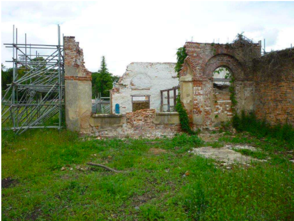
South elevation of south wing – 2022
