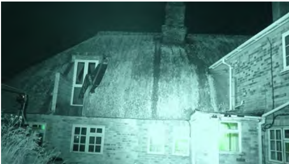
Figure 3: Still from infrared camera facing the northeastern and northern elevations.
