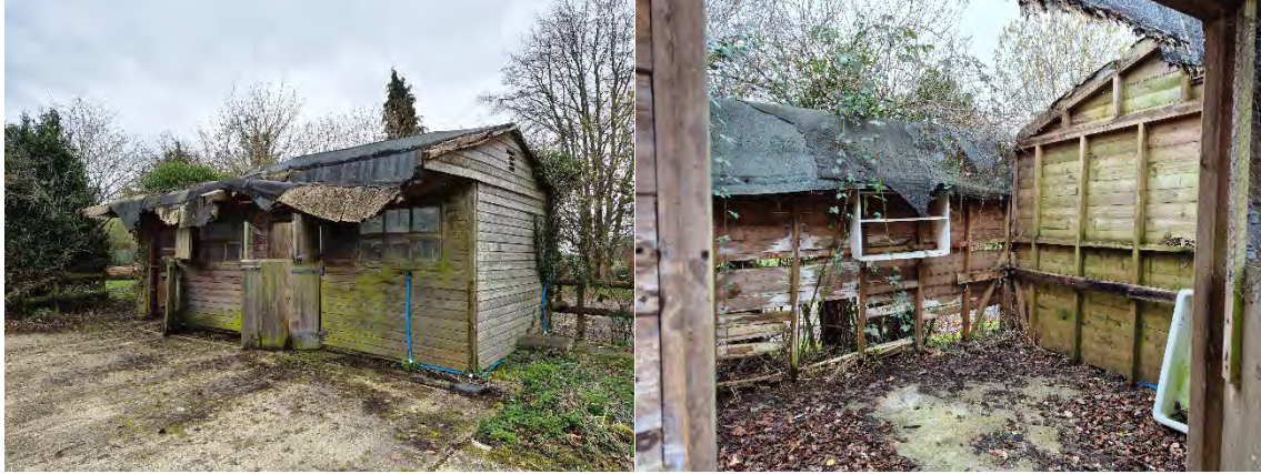
Figure 21: External view of the Stable building Figure 22: Internal of the Stable building
