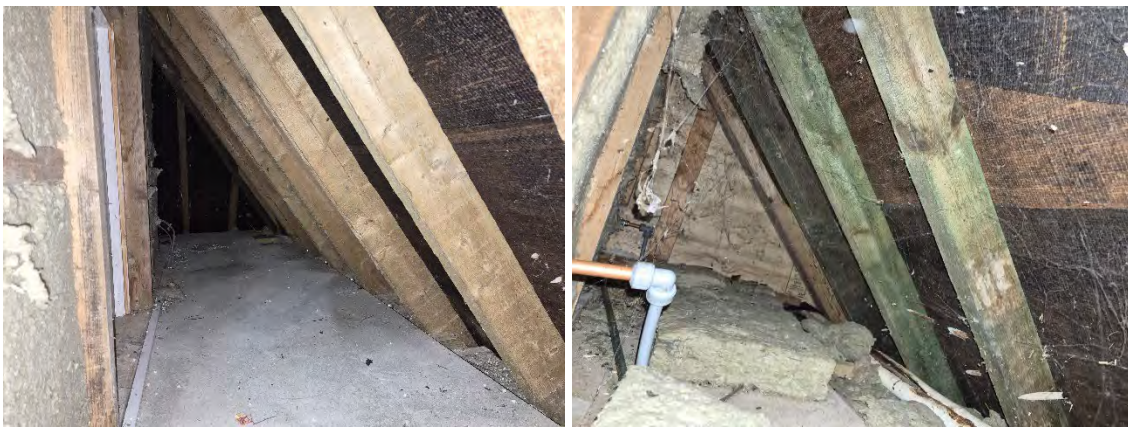
Figure 16: Internal view of southeastern eaves Figure 17: Internal view of flank void with insulation material
