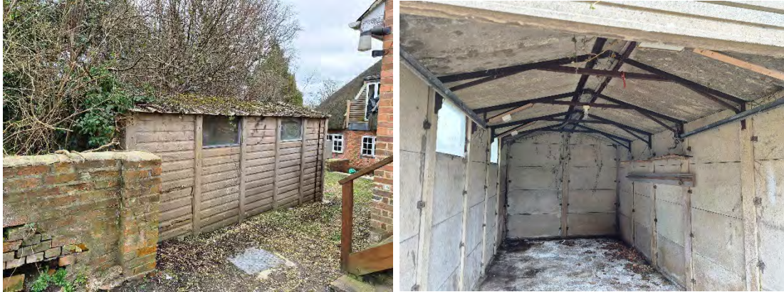
Figures 18 External view of the concrete garage. Figure 19: Internal view of the concrete garage.
