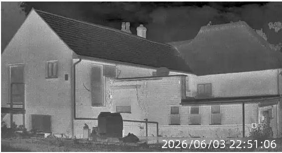
Figure 1: Still from thermal camera facing the Northwestern elevations.
