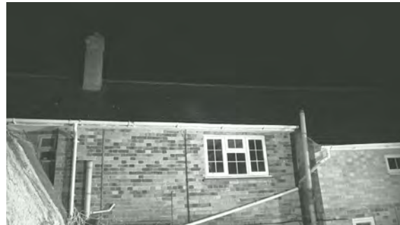
Figure 4: Still from infrared camera facing the northern elevations.
