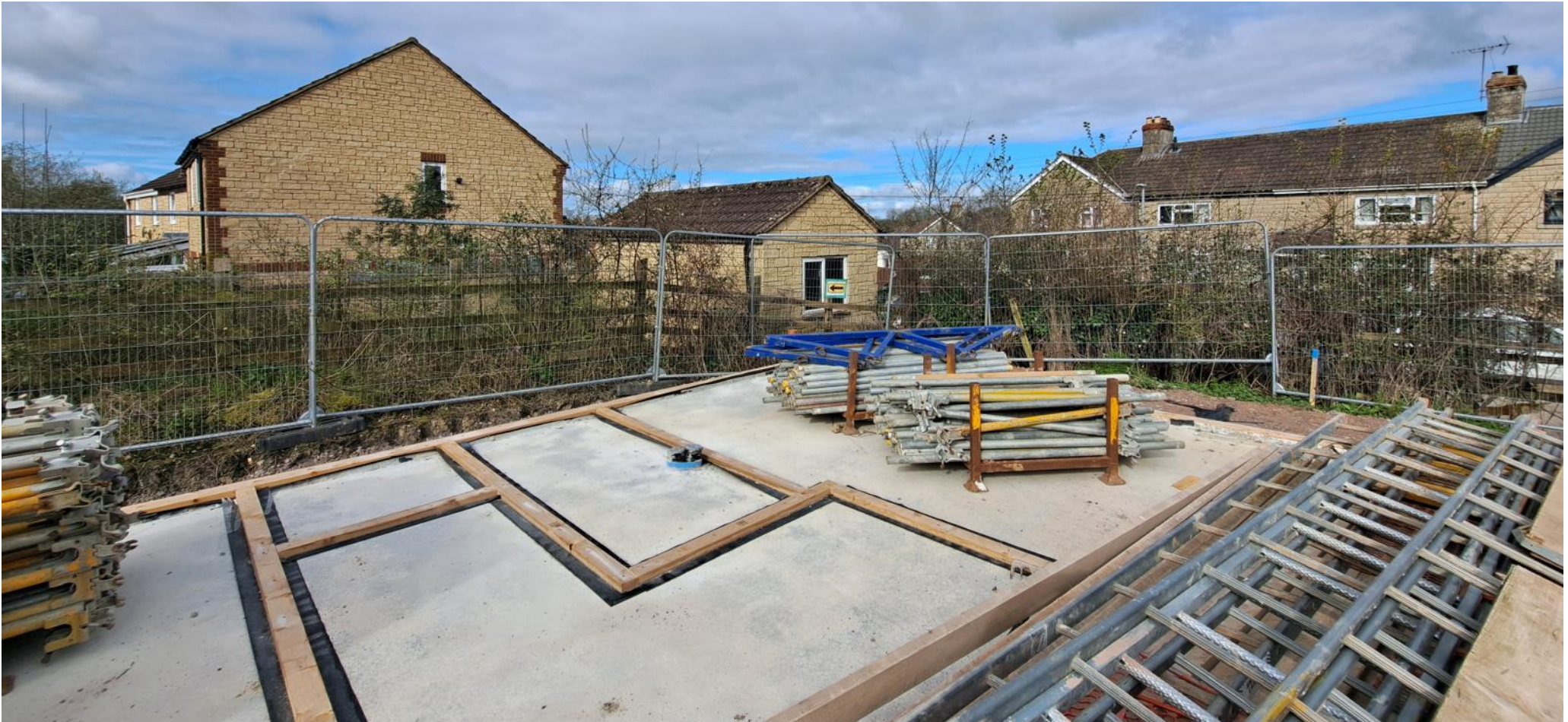
Photo 2: showing the sparse existing hedgerow that forms the shared boundary with No. 12 Low Lane, which is proposed to be replaced with a 1.8m close boarded fence. The woody planting that was intended to be planted to augment the existing hedge will be planted in the area of public open space to ensure no net change to the agreed BNG mitigation.
