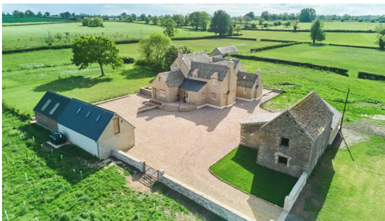
Figure 3: Host dwelling, outbuilding and barn (bluebook)
