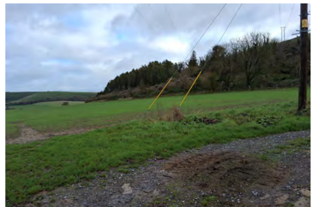
Plate 8. View east along cable route from Ferne Hollow. (ST 93282 21230)
