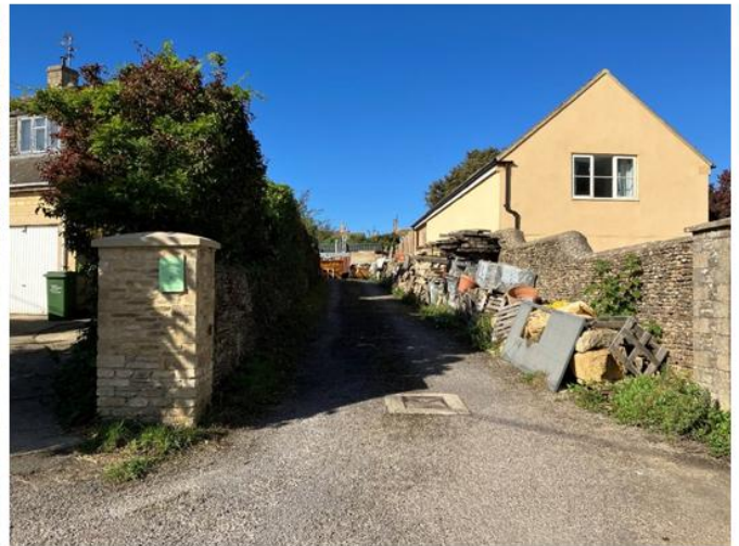
Access to the builder's yard / annex building of no.4 Grove Road
