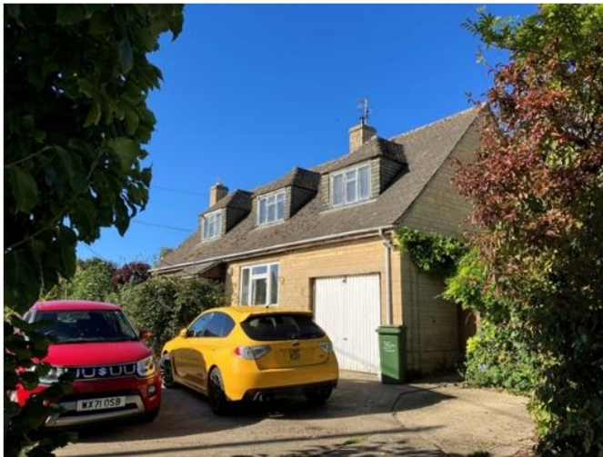
Existing no.5 Grove Road
