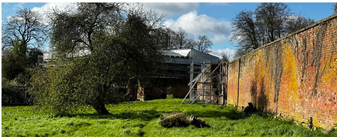
Figure 8 – View towards South with Outer Garden Wall to the right and Old Stables in the background
