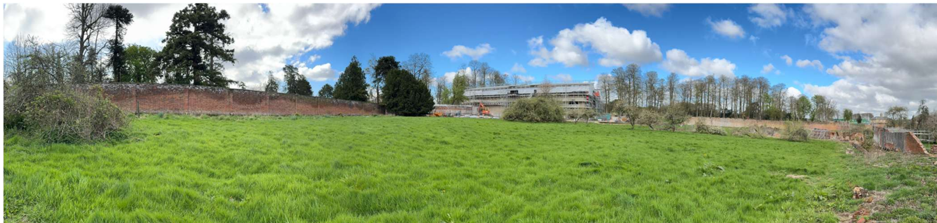
Figure 4 - Panorama view towards the Old Stables, East Garden Wall and remains of Spine Wall & Building 16
