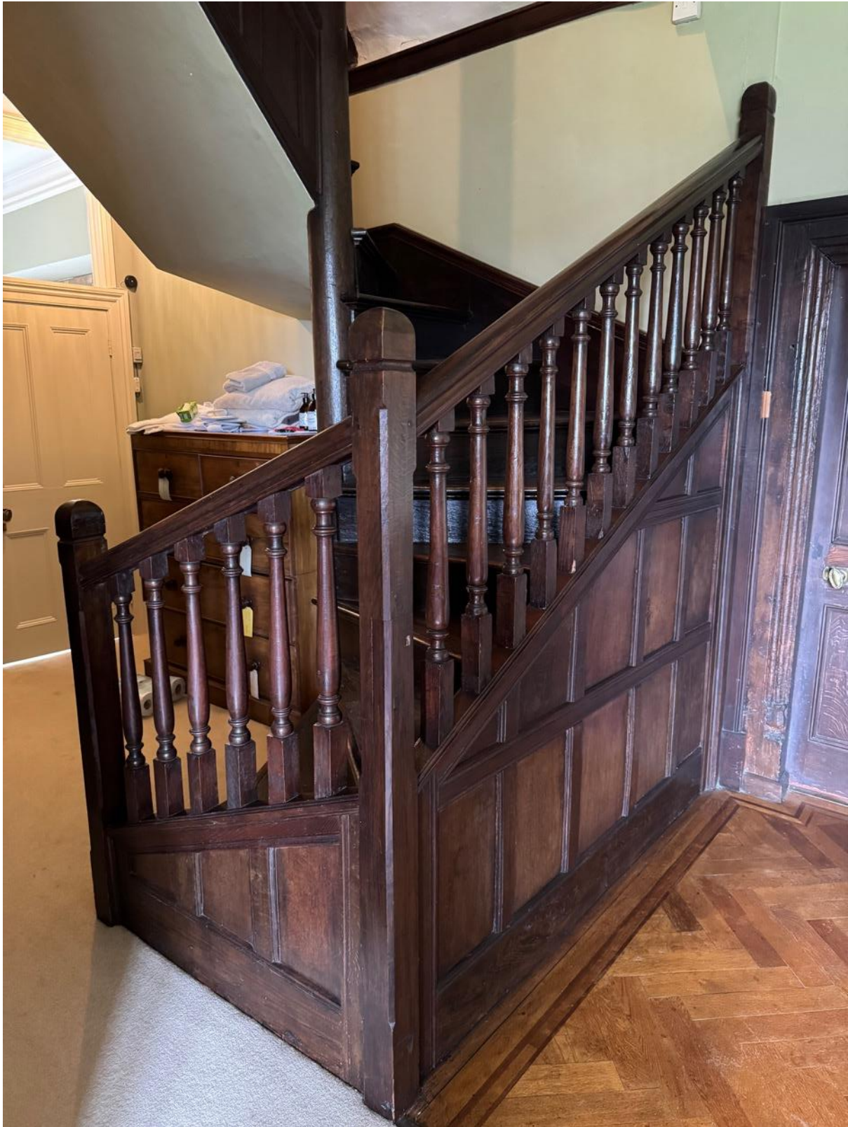
Figure 15: Probably 17 th century winder stair from first to second floor
