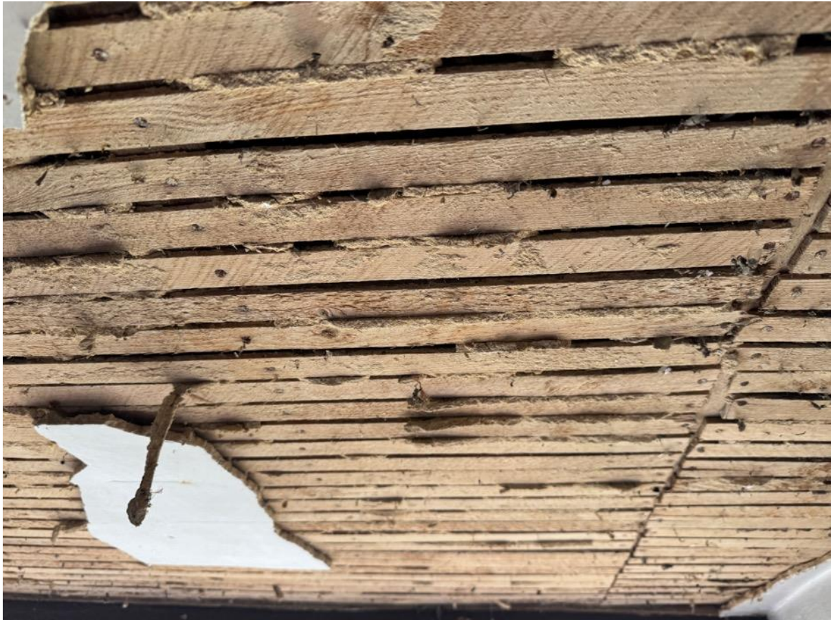
Figure 29: Sawn laths to ceiling of dormer window to south-west wing
