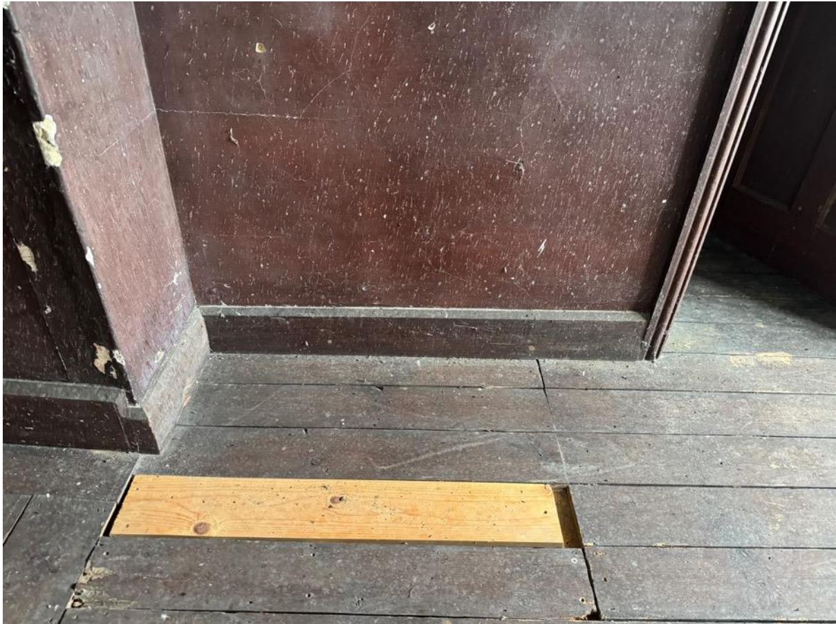
Figure 27: Narrow softwood boards – in the area proposed for the new staircase (in front of the door pictured)
