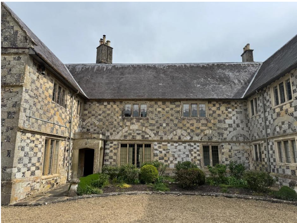
Figure 2: West elevation - series of blocked openings with relieving arches above
