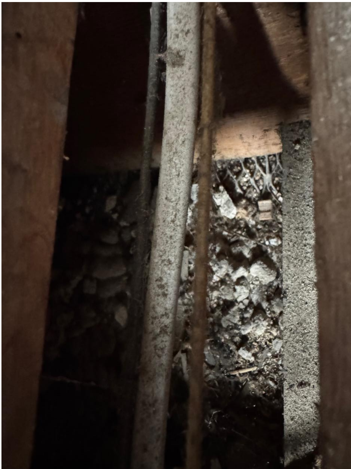
Figure 28: Photo taken between the joist showing metal gauze make-up of ceiling to first floor.
