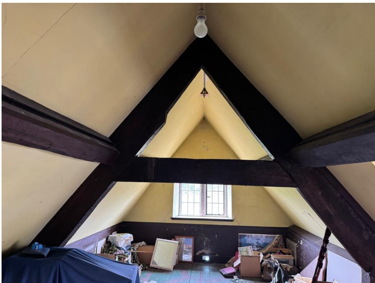
Figure 20: Straight collar to remaining truss to north-west wing
