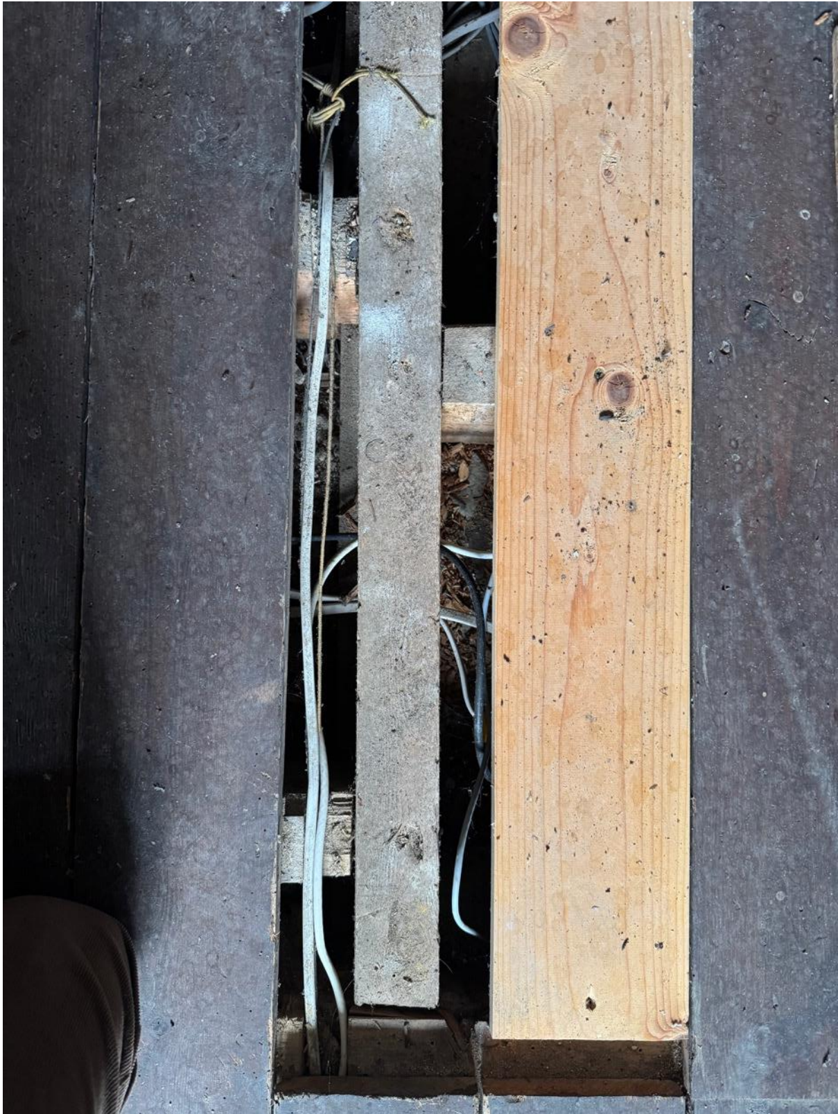
Figure 30: Sawn softwood joists in area of floor proposed for staircase installation
