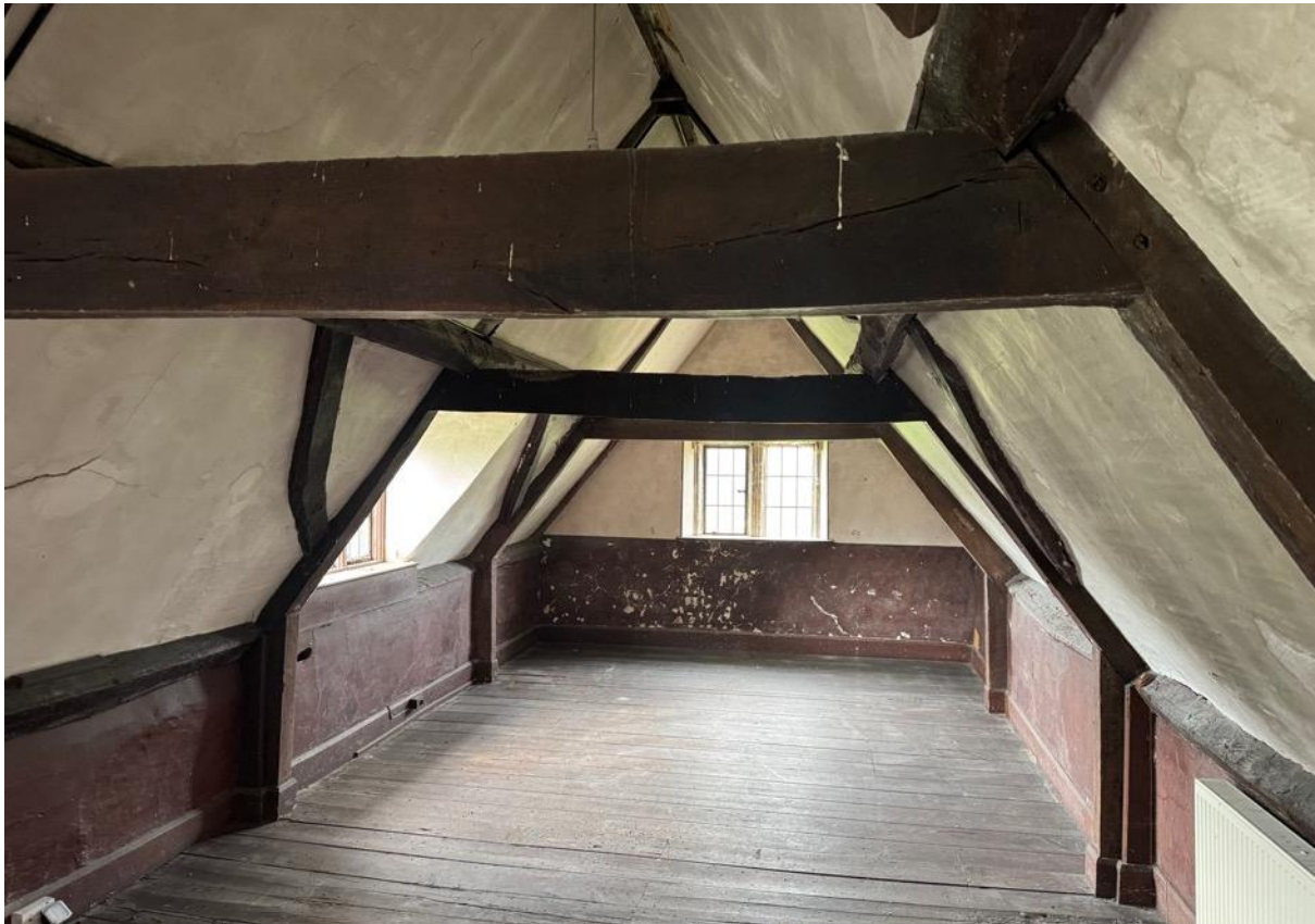
Figure 22: Roof structure to south-west wing- clapsed purlins and straight collars, but with straight wind braces
