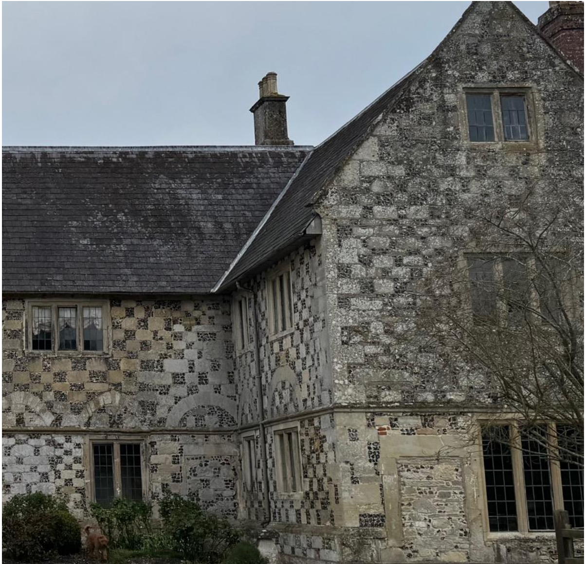
Figure 4: Change in stone work between west elevation and south-west wing
