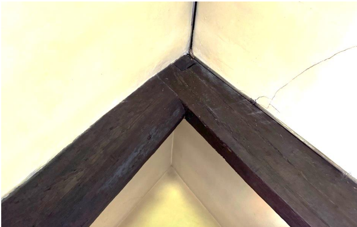
Figure 19: Evidence for a ridge purlin – suggesting early date for this truss (and its neighbour)
