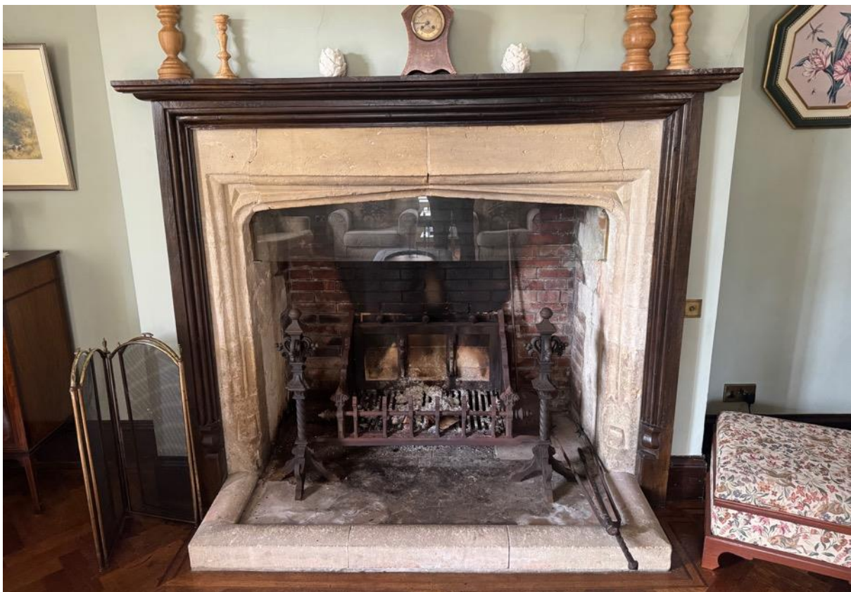
Figure 12: Drawing Room: Late 16 th / early 17 th century fire surround – vase stops and ovolo and hollow moulding
