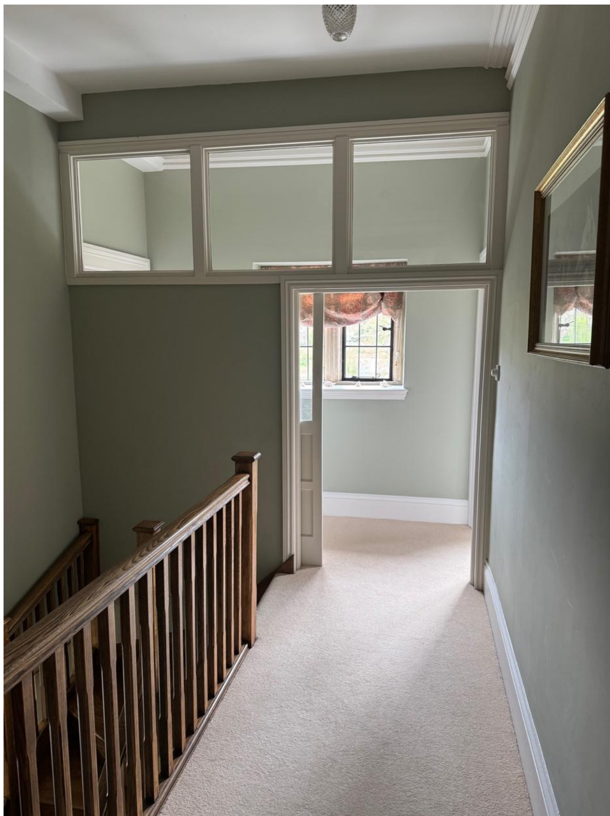
Figure 26: New partitions to first floor (allowing access to the bathroom)
