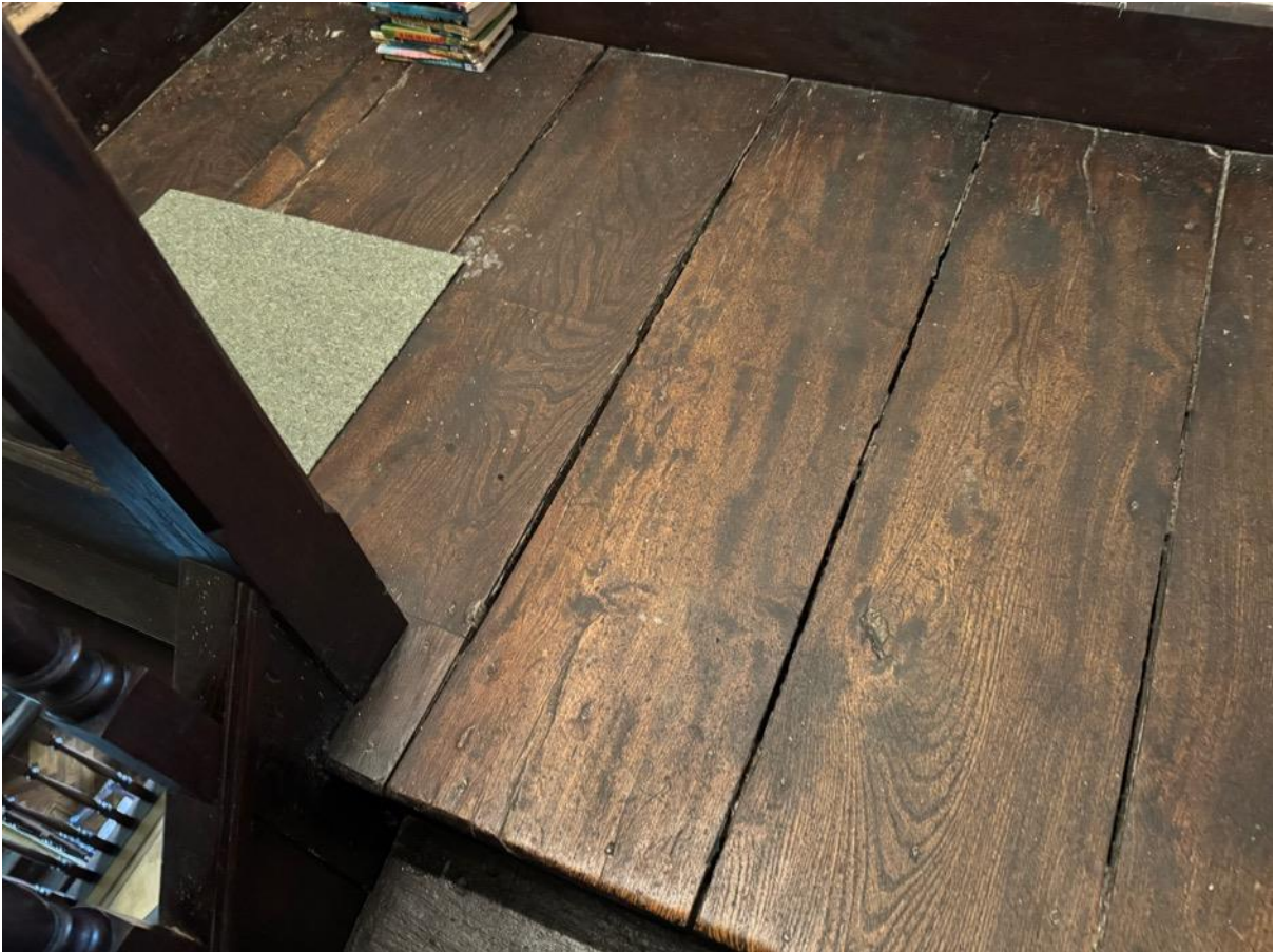
Figure 16: Oak boards to landing of winder stair
