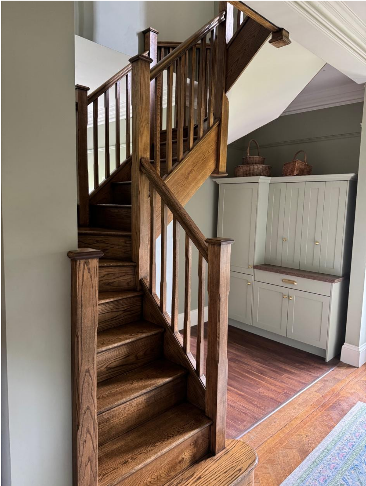
Figure 25: The staircase from ground to first floor has already been constructed
