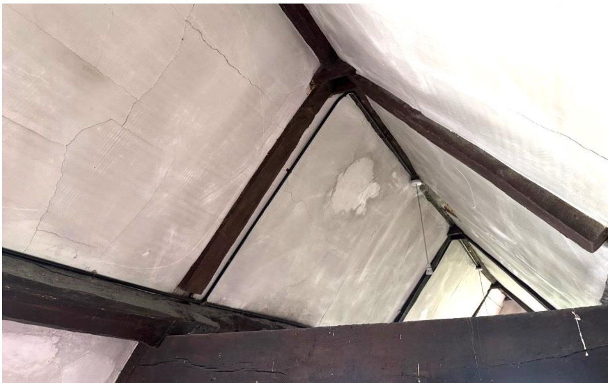
Figure 23: Yolk to ridge-piece (often an 18 th century feature)
