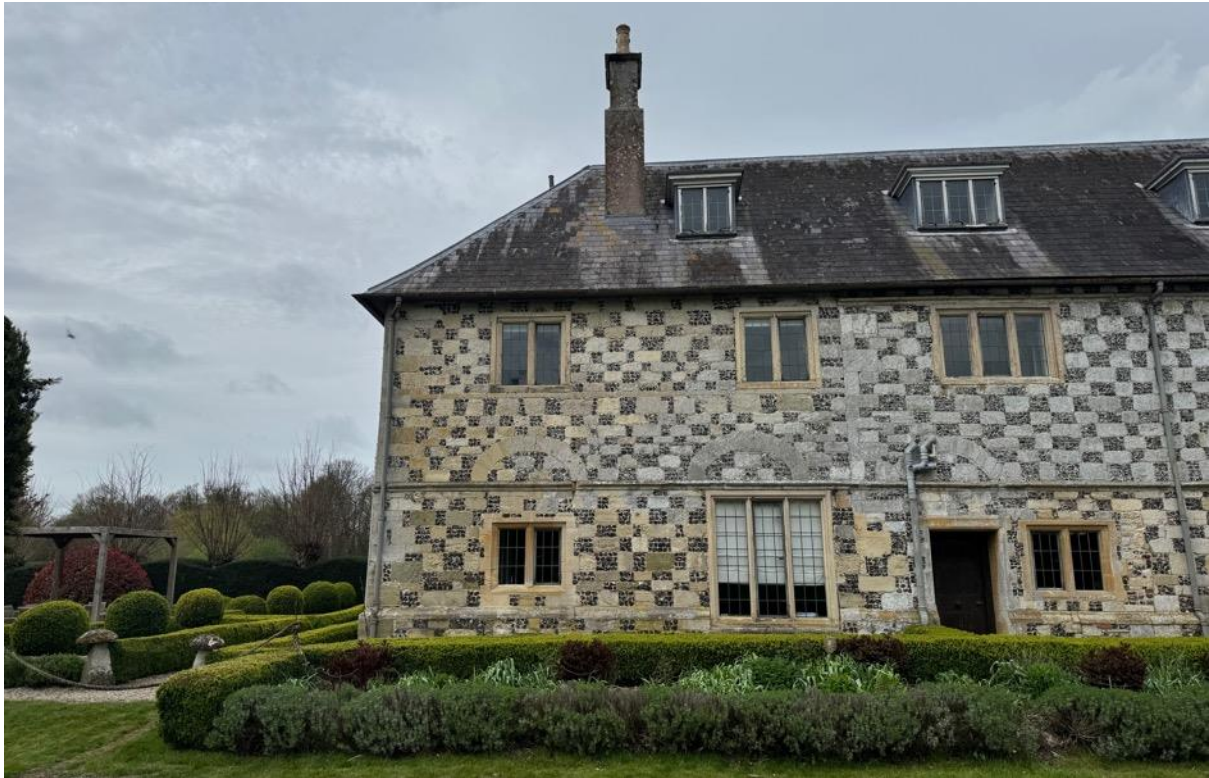
Figure 7: Straight joint to stonework between bays 2 and 3
