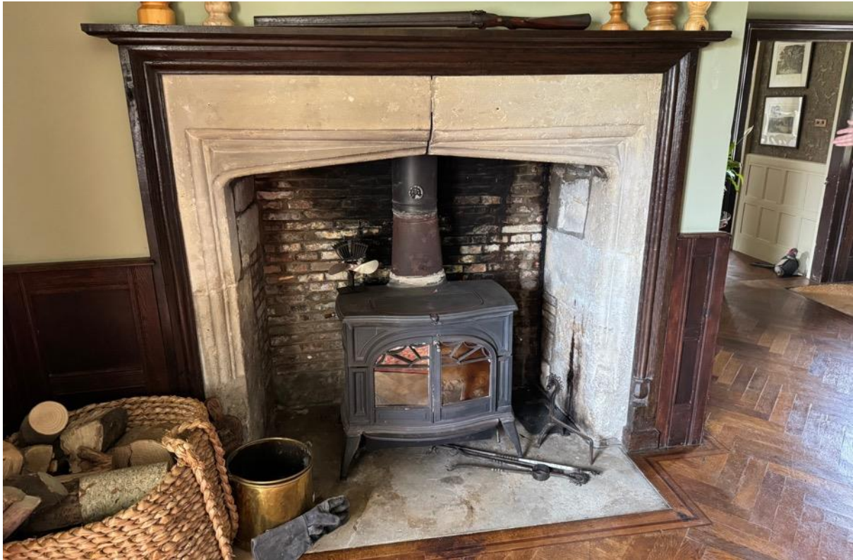
Figure 11: Late 16 th / early 17 th century fire surround to hall – vase stops and ovolo and hollow moulding
