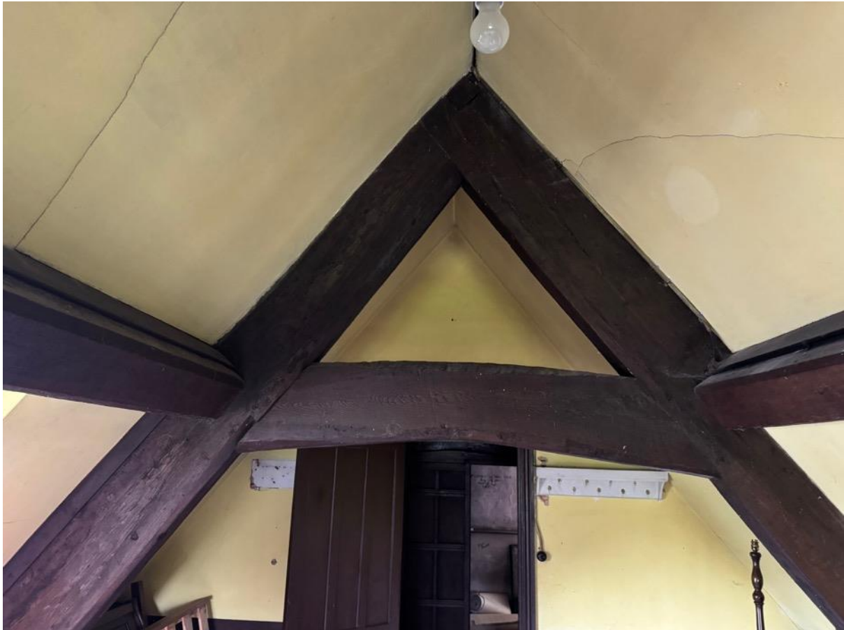
Figure 18: Roof structure of two bay of north-west wing – possibly early 16 th century?
