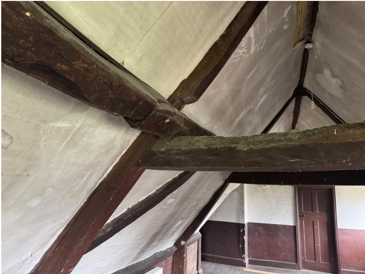
Figure 24: Purlins are re-set (the cut out to the principal rafter is much larger (consistently) than the present purlins
