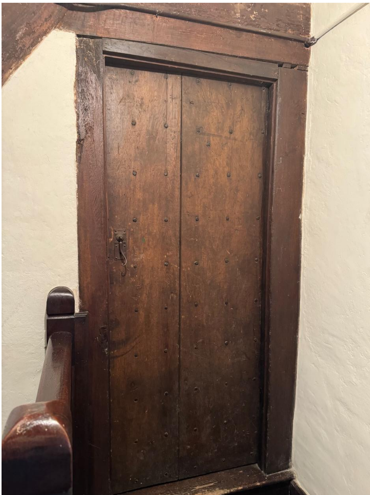
Figure 17: 17 th century door at north side of winder stair lobby
