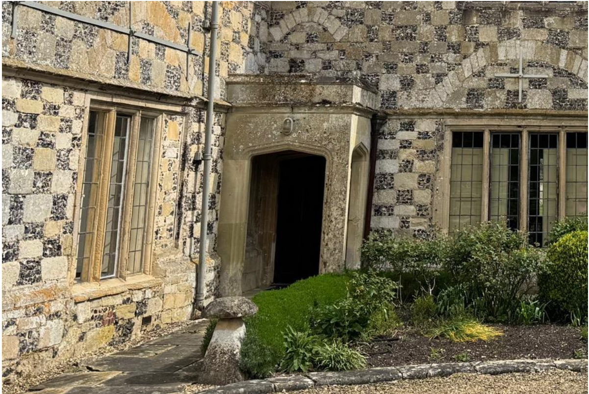
Figure 9: Stone porch entrance (west elevation)
