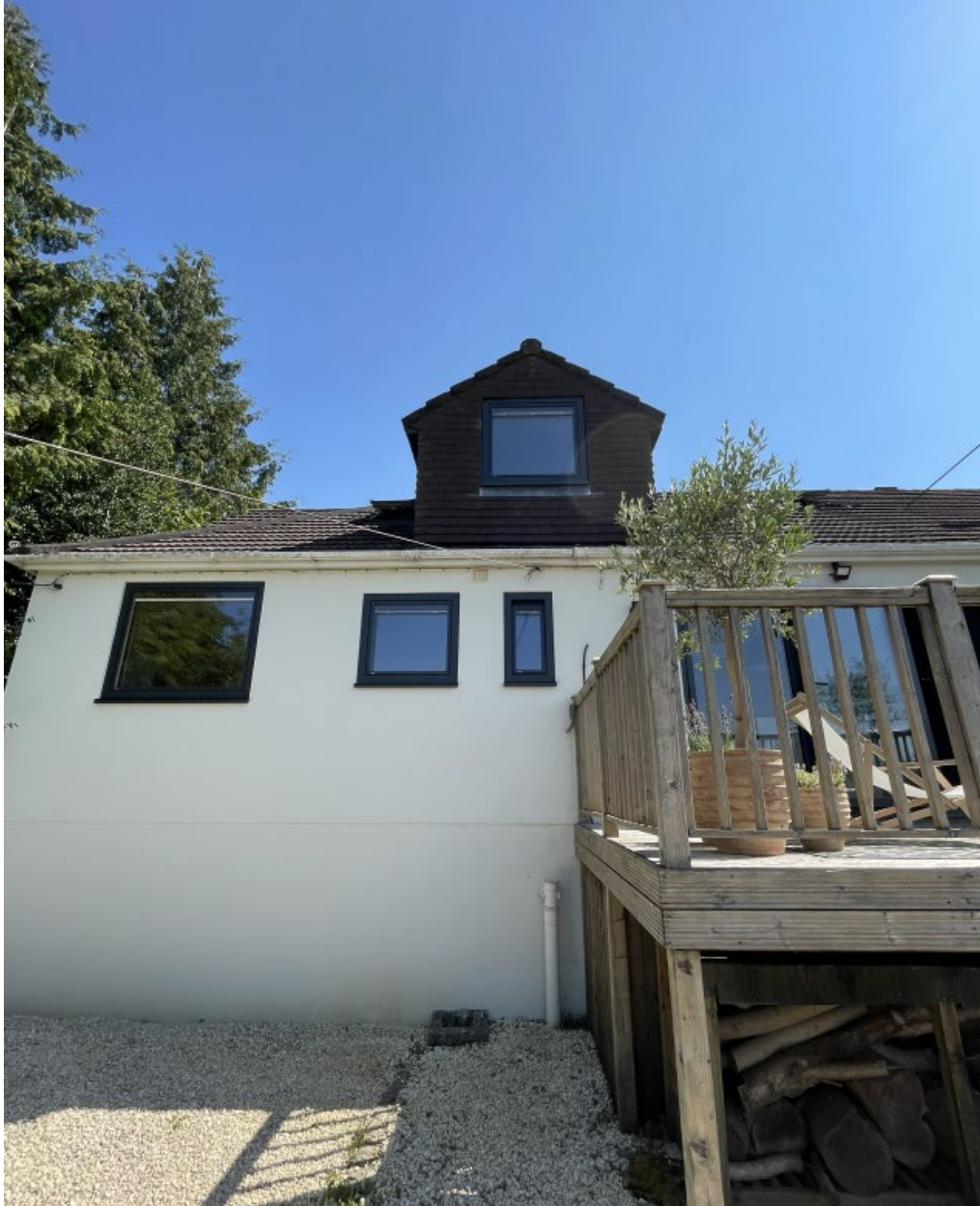
Fig. 2 – Part rear elevation of property.
