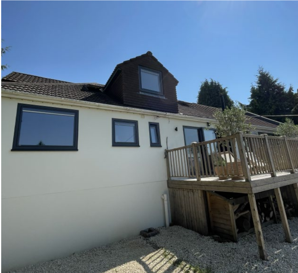
Fig. 3 – Rear elevation of property.
