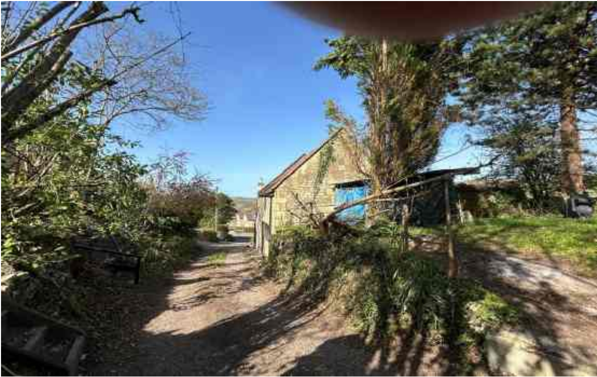
View towards Devizes Road with Blacksmiths Cottage on the right
