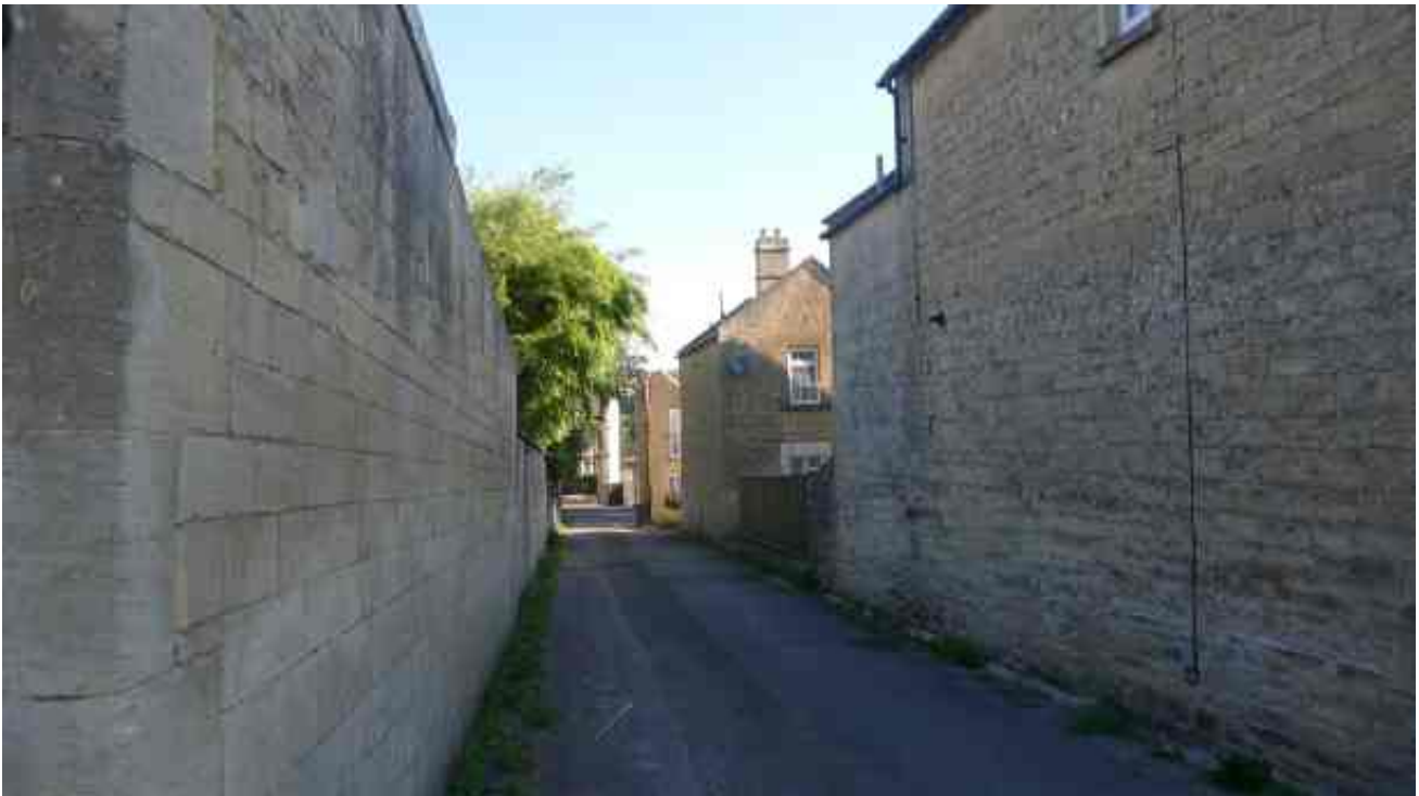
Burtons Lane (observe narrowness and window juxtaposition)
