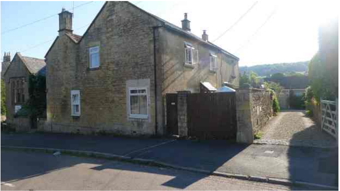
Chapel Lane (house abutting footpath which also overlooks neighbour)
