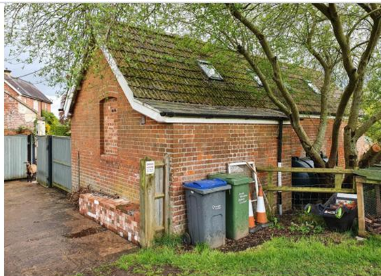
Figure 5 - West and north elevations of spa outbuilding
