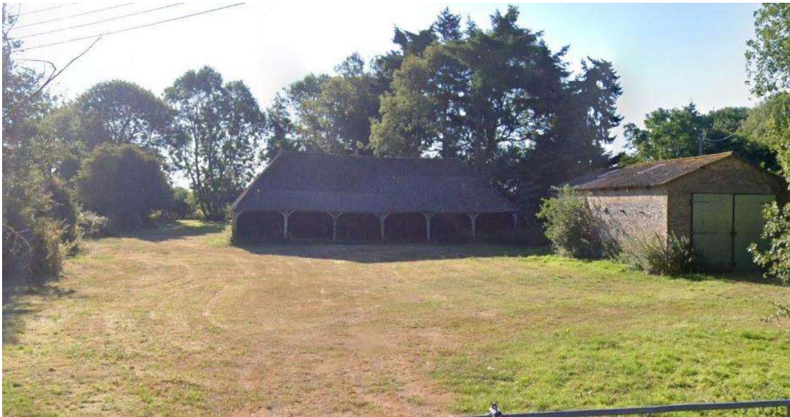
View of the Goat Barn seen from the site access, looking east.
