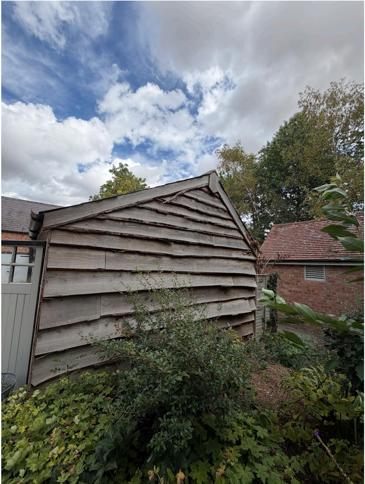
5 - Southern elevation of the garage showing surrounding garden
