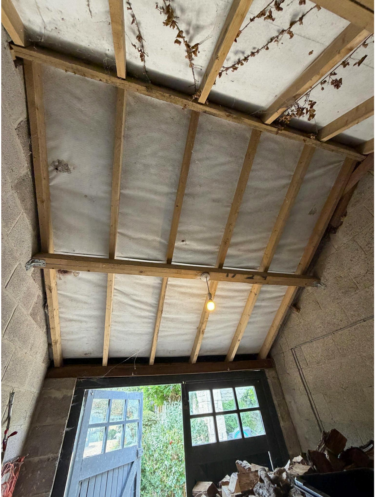
14 - Garage roof looking towards the entrance
