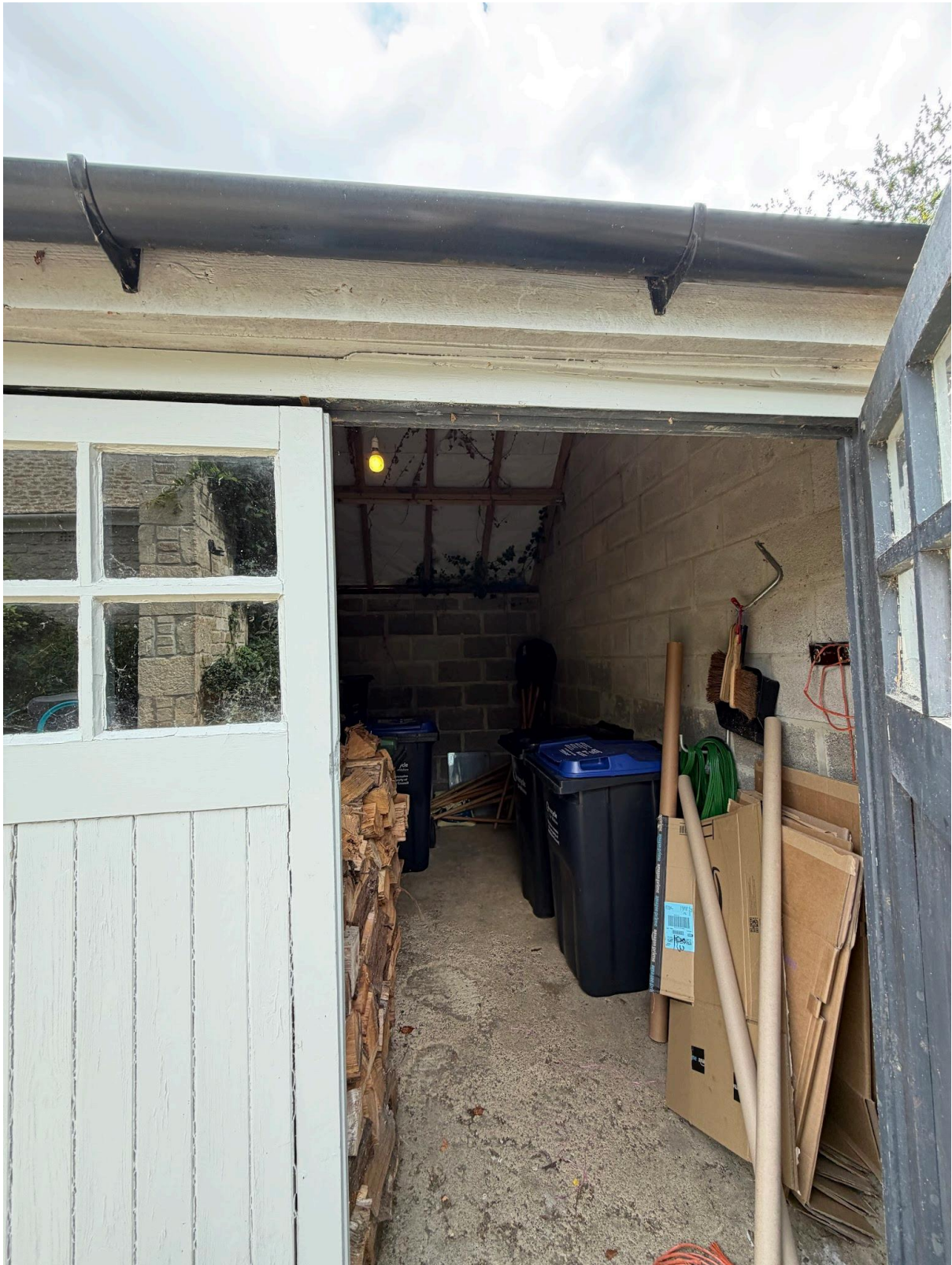
6 - Entrance to garage from Western elevation
