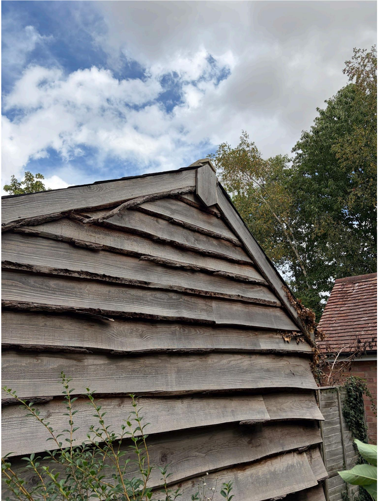
4 - Southern elevation of the garage showing slight lifting of the cladding with no visible signs of bats
