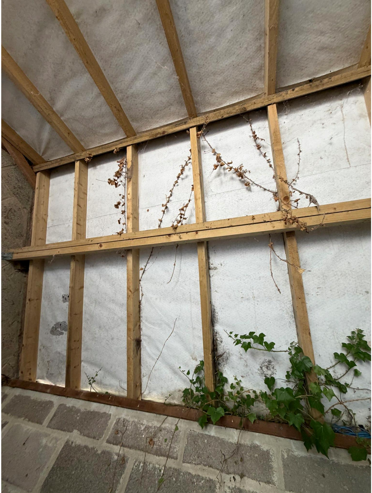
9 - Garage roof meeting Eastern elevation showing small opening and Ivy
