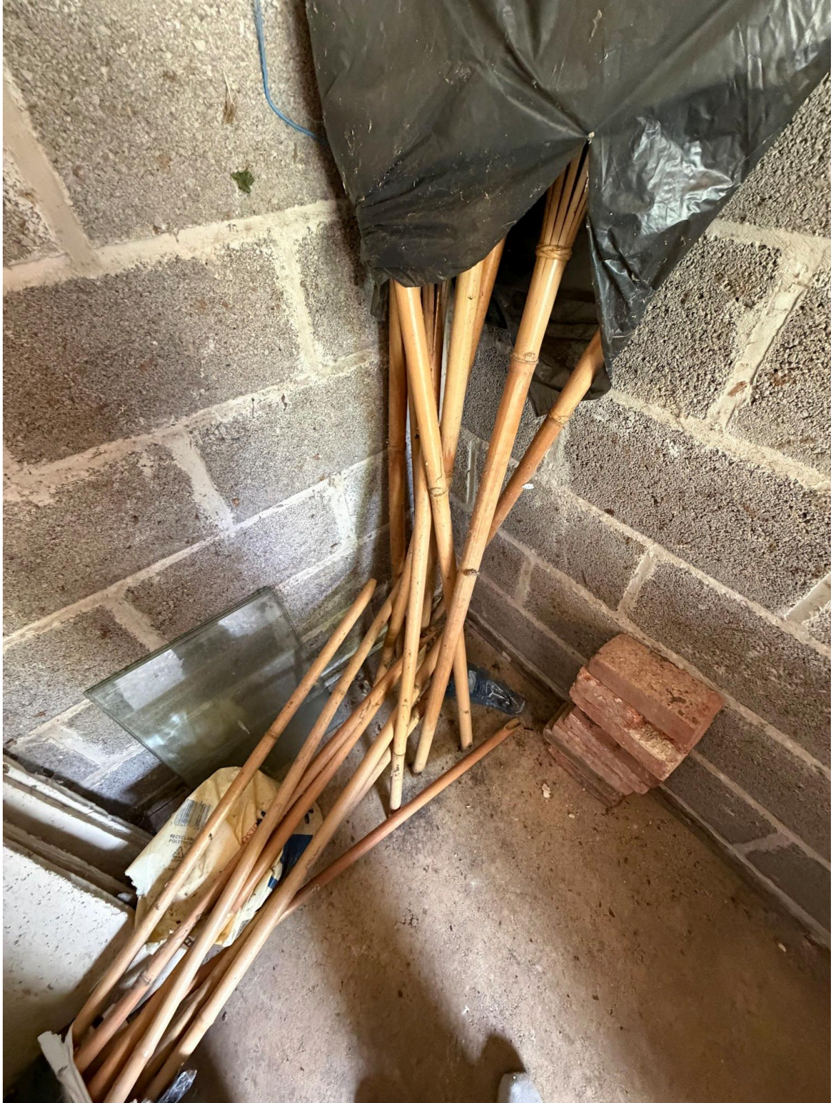
10 - Garage floor with no visible signs of bats
