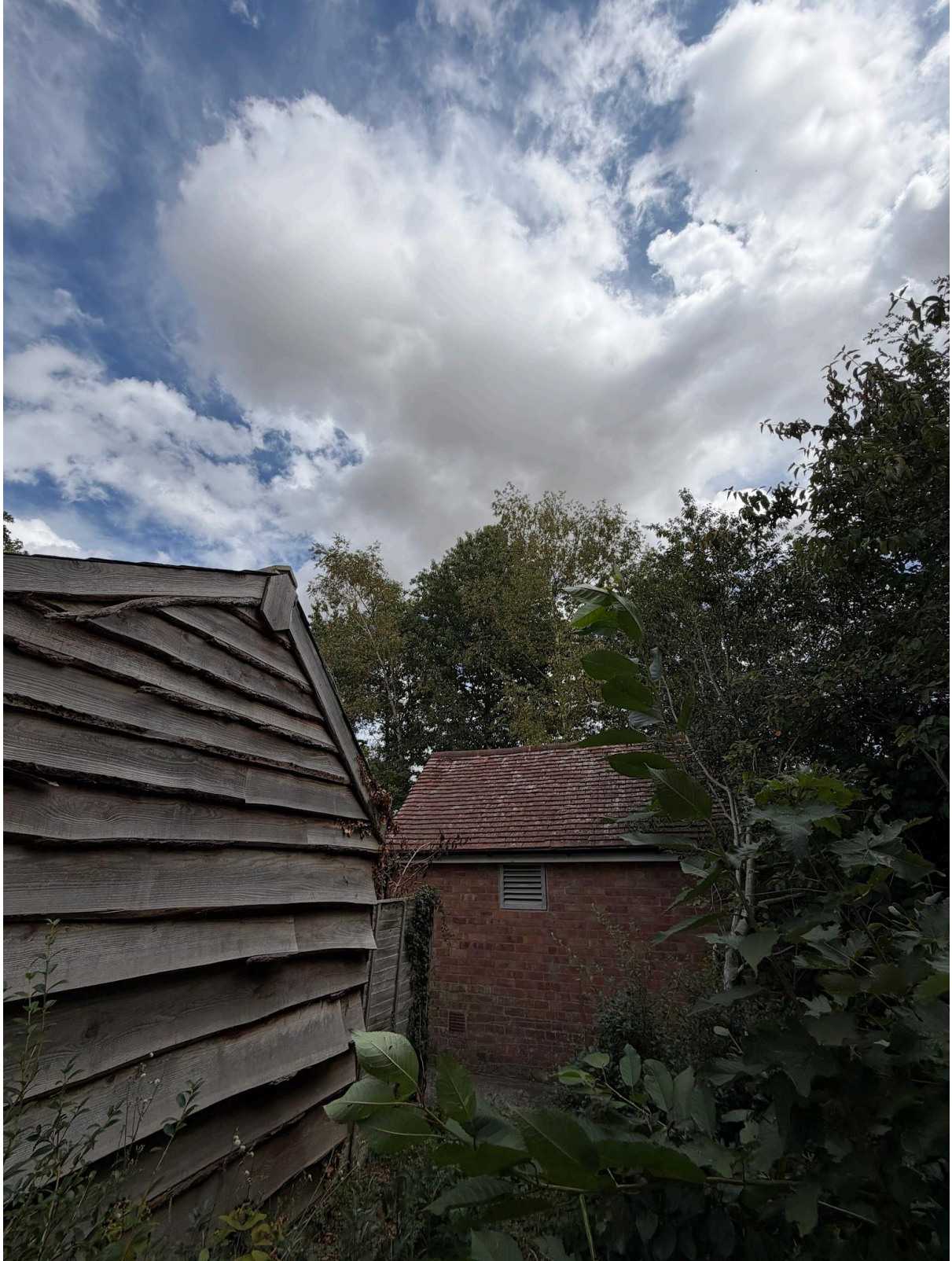
3 - Southern elevation of garage showing slight lifting of the cladding with no visible signs of bats
