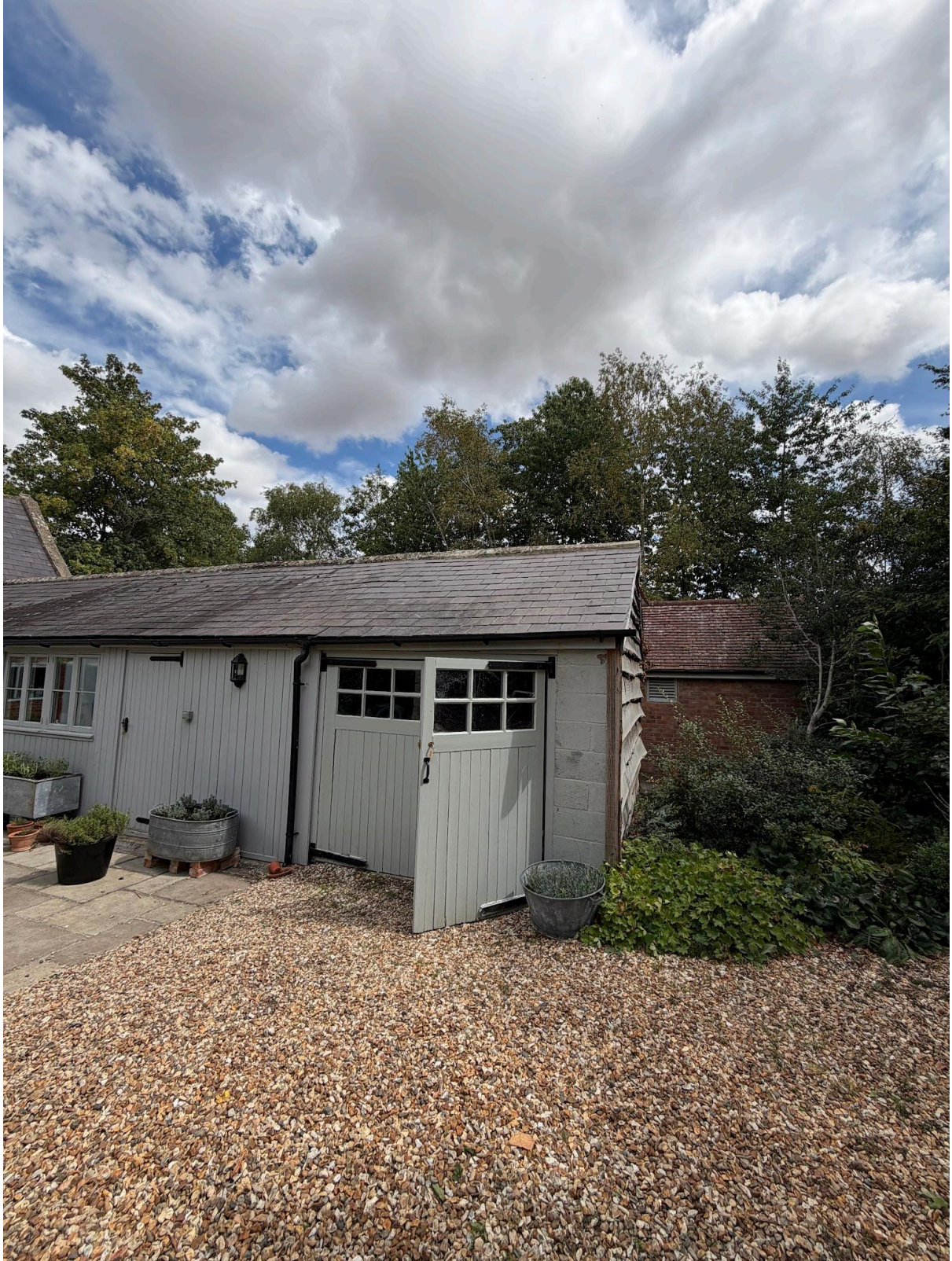
15 - Exterior of garage showing no lifting roof tiles
