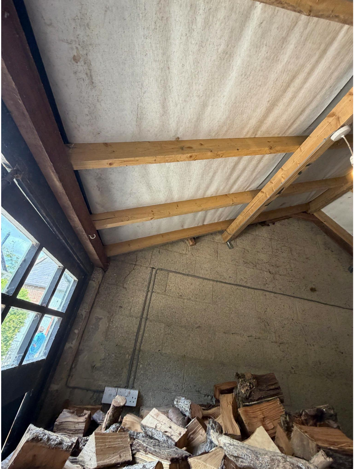
11 - Internal Northern elevation of garage
