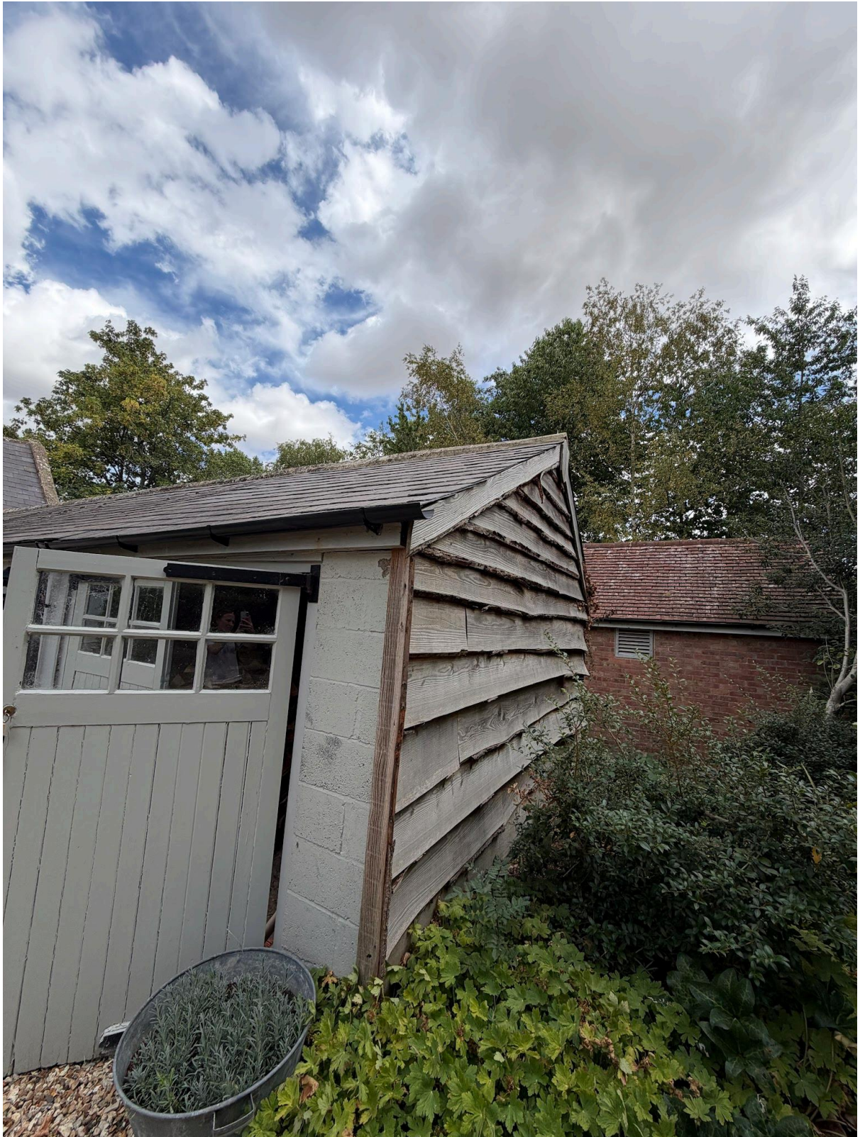
2 - Southern and Western elevation of the garage showing wooden cladding
