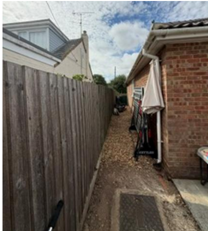
Fence between Bourne Villa and Martinsgate – taken from Bourne Villa
