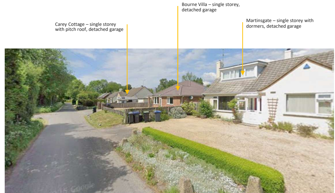
Street view looking west
