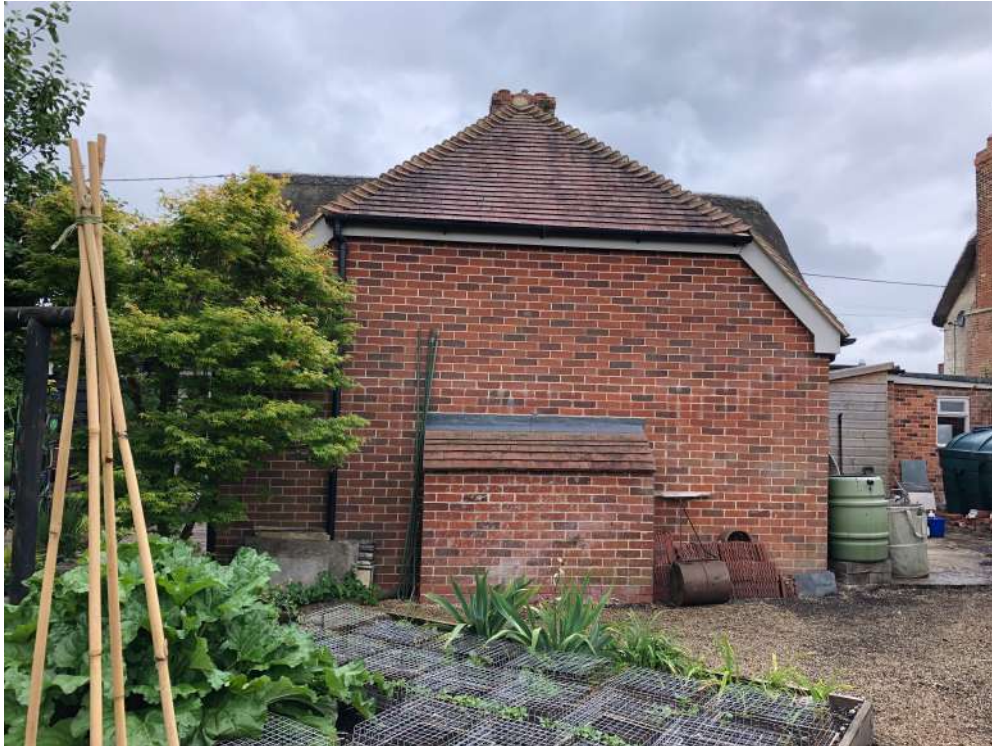
View of 2006 extension (left) and 1970's extension (right) from garden
