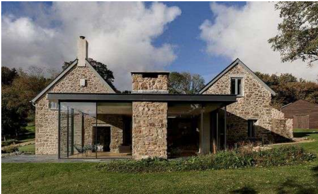
West Yard Farm, van Ellen and Sheryn – Example of slim framed glazing allowing views through to existing historic building
