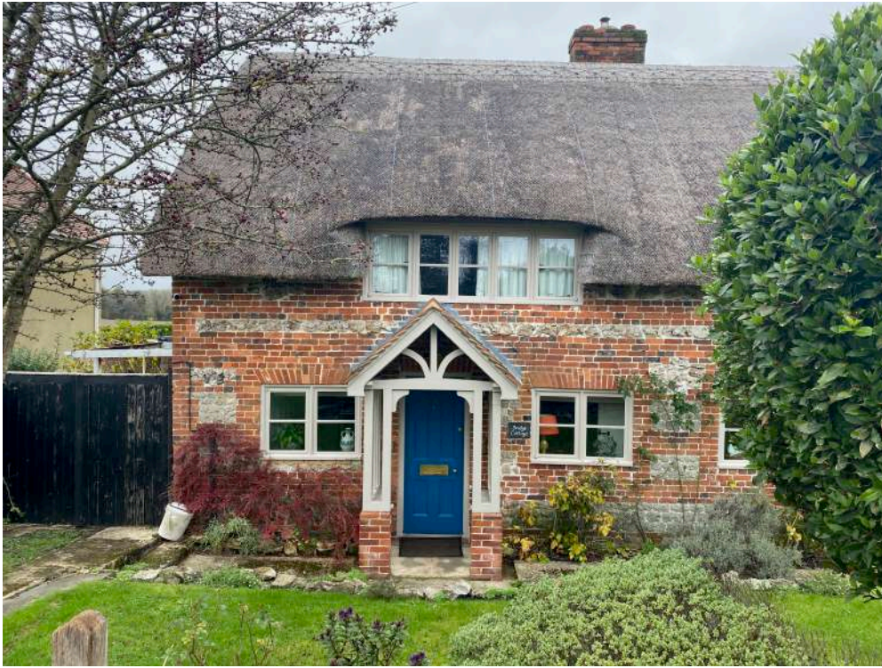
View of original house from Alton Road
