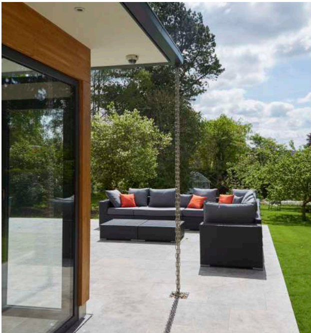
Example of a rain chain
