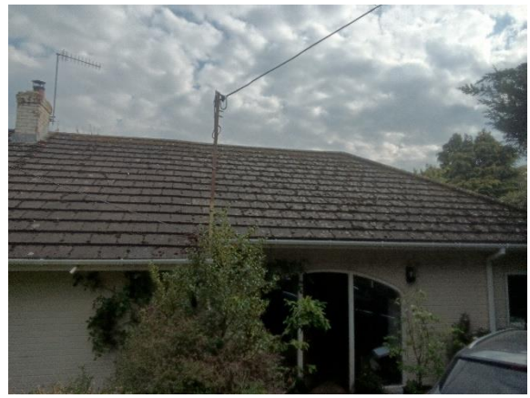
Plate 2. Front elevation of B1.
