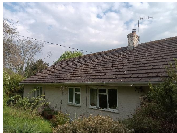
Plate 1. Rear elevation of B1.
