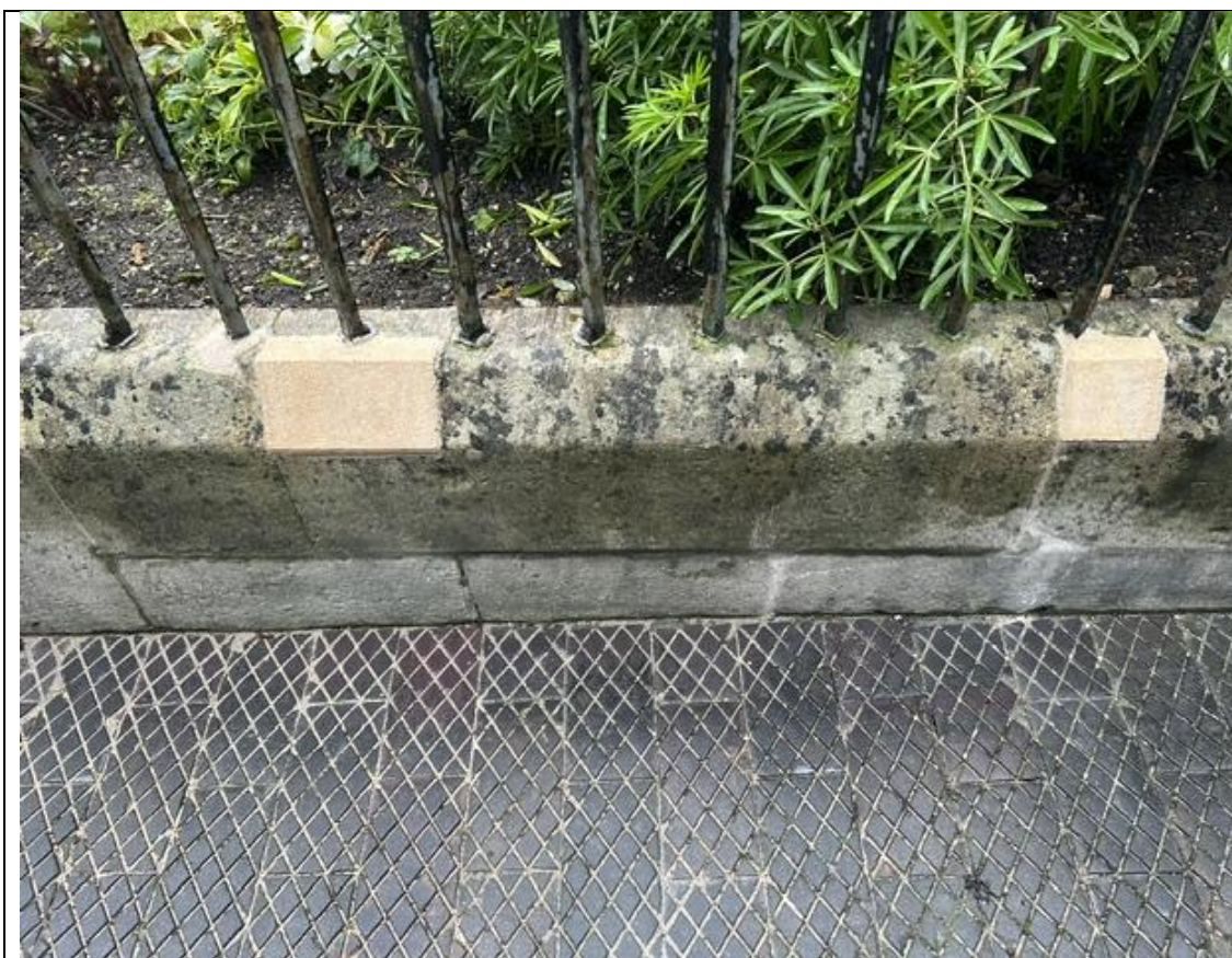
Fig 4. Photo of small indent repairs to side railing plinths using matching stone and lime mortar.
