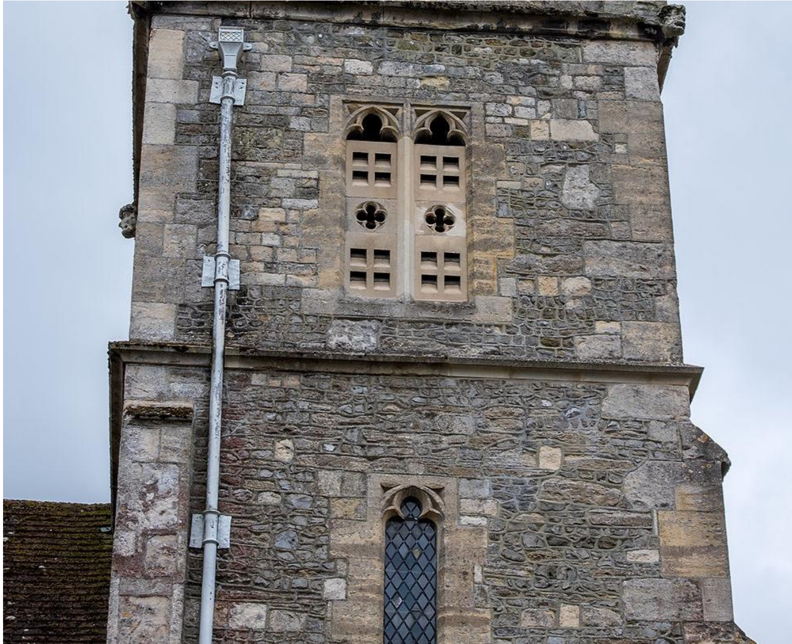
Continued repainting of the downpipes
