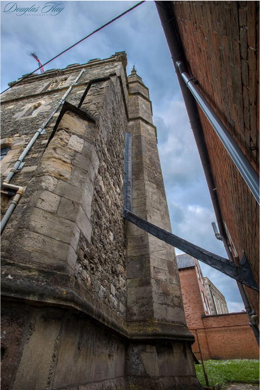
Repairs to the lead bell rope shoot
