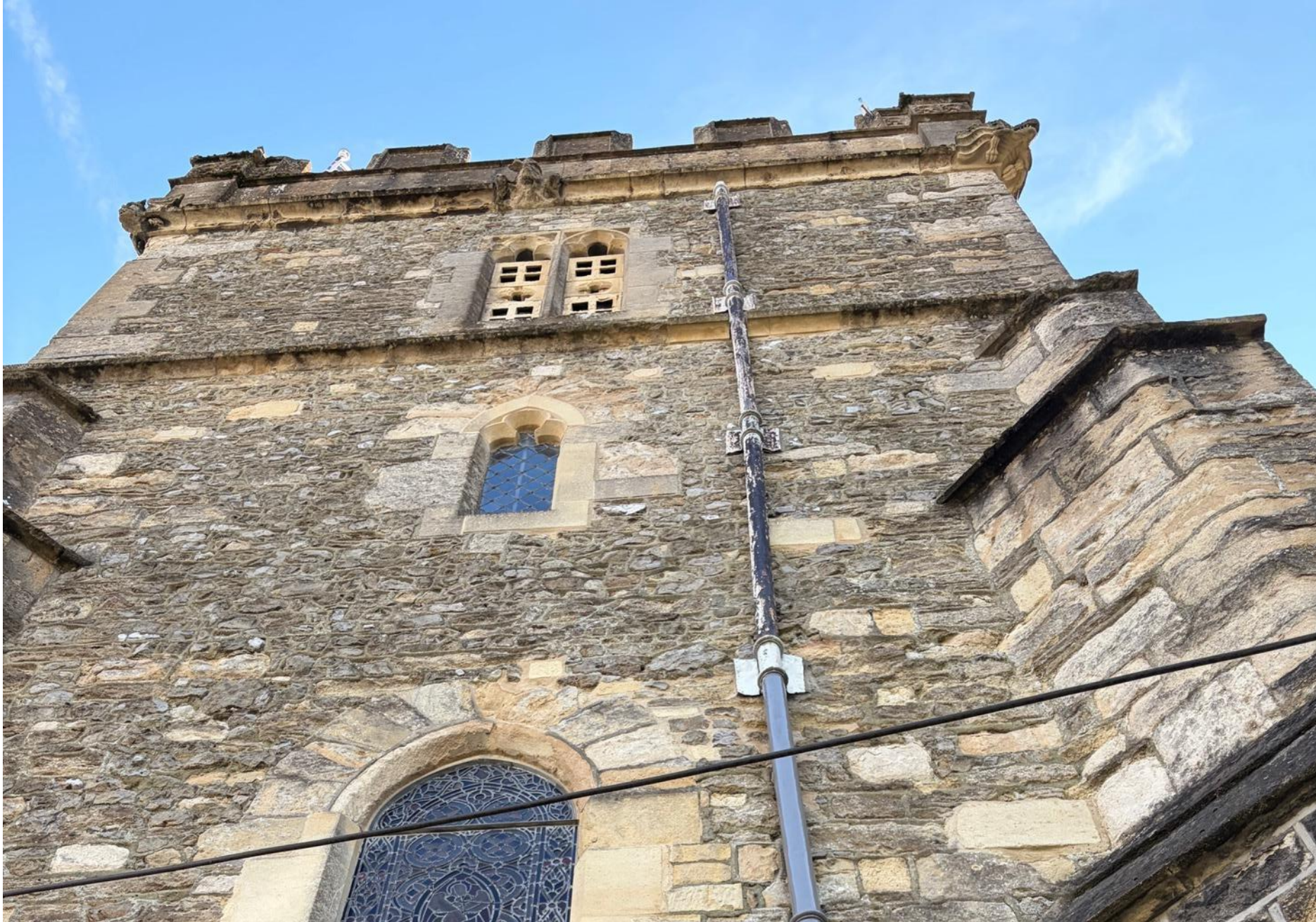
Continued repainting of the downpipes
