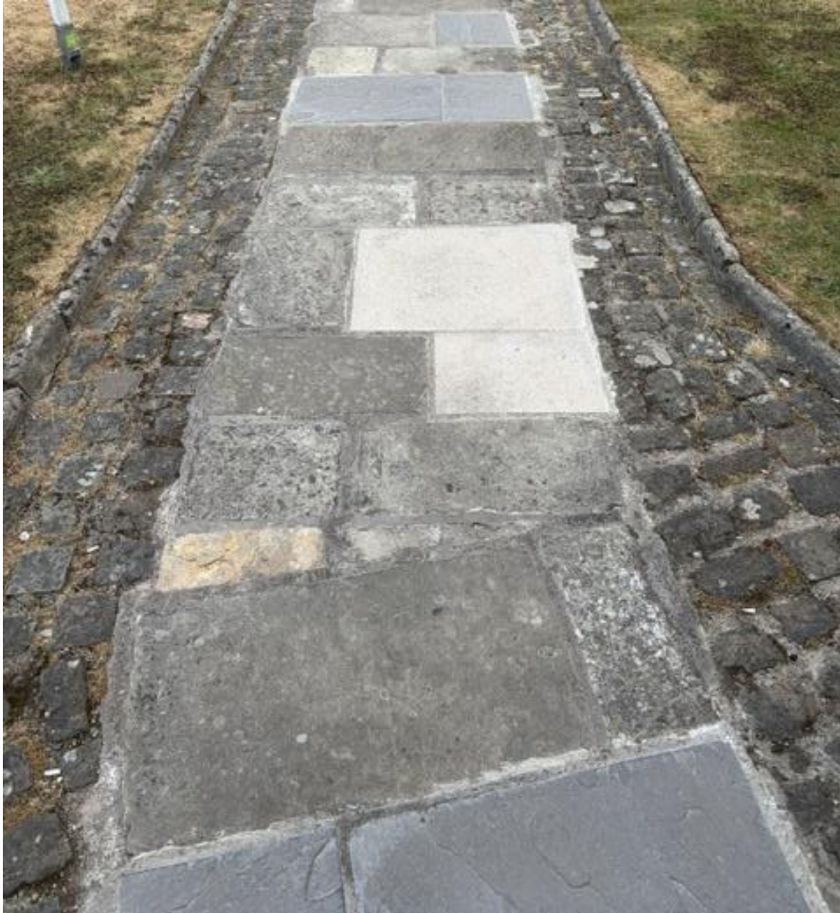
Chapel path repointing
