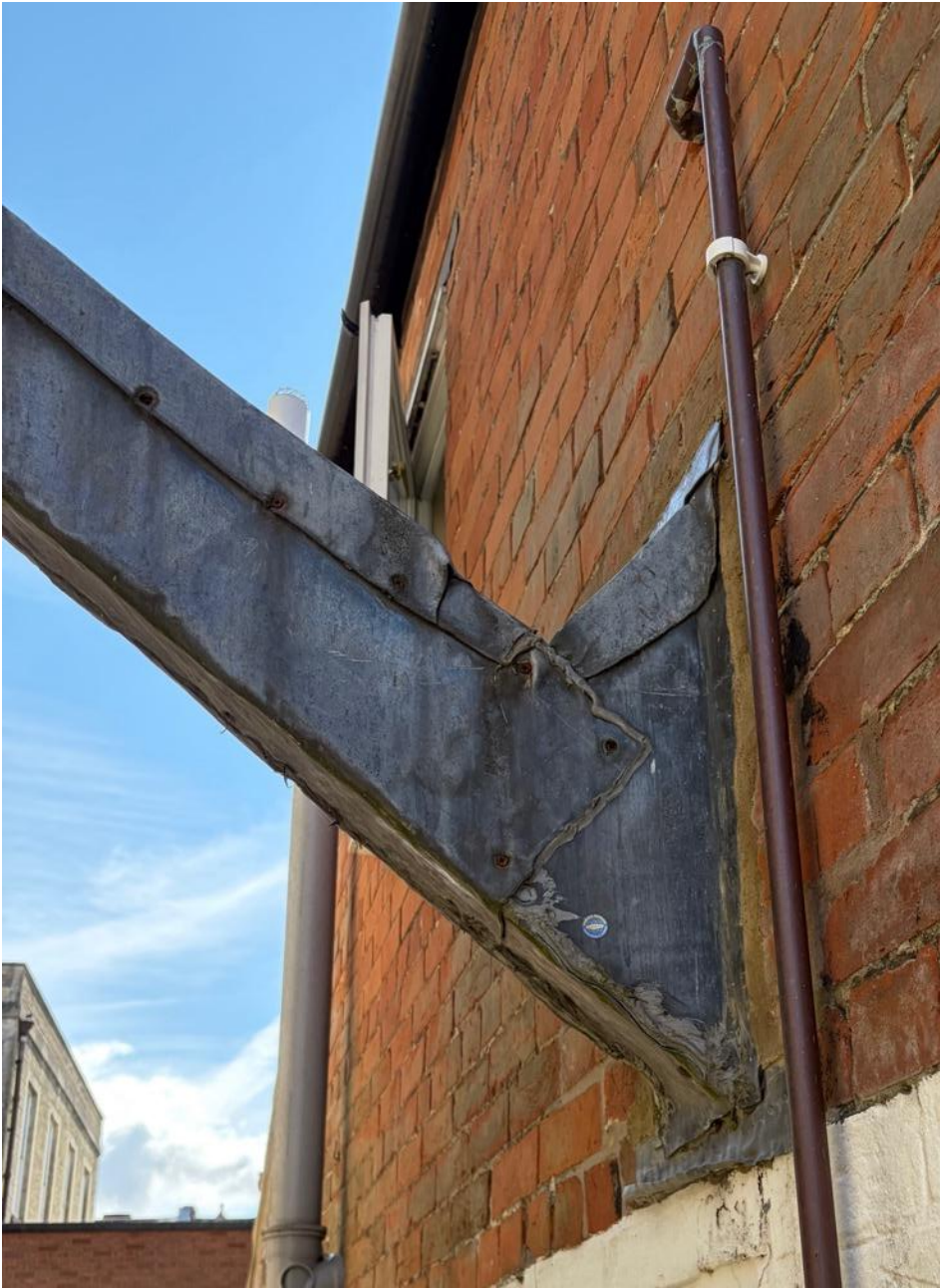
Repairs to the lead bell rope shoot
