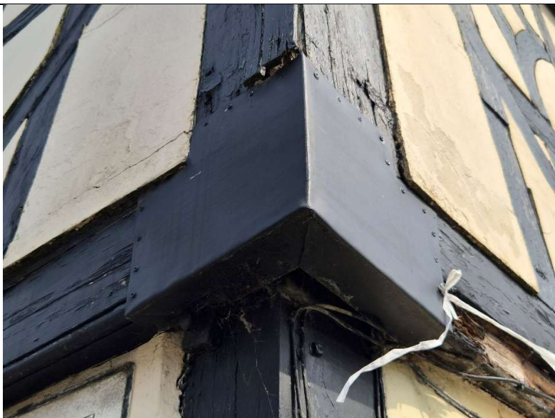
3. uPVC cover strip to south corner of building
