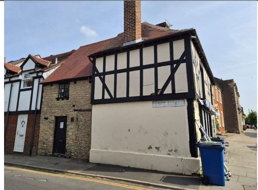
2. Gable end elevation, showing frontmost part of the building, together with the rear 'extension'.
