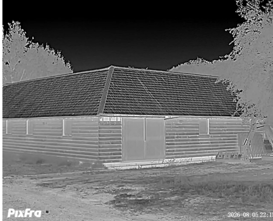
Figure 2: Northwestern elevation of the stable.
