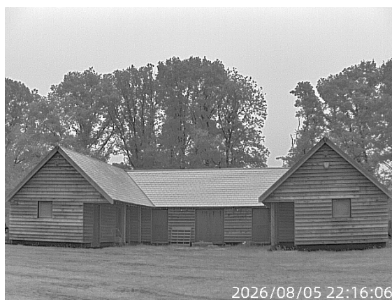
Figure 1: Southern elevation of the stable.
