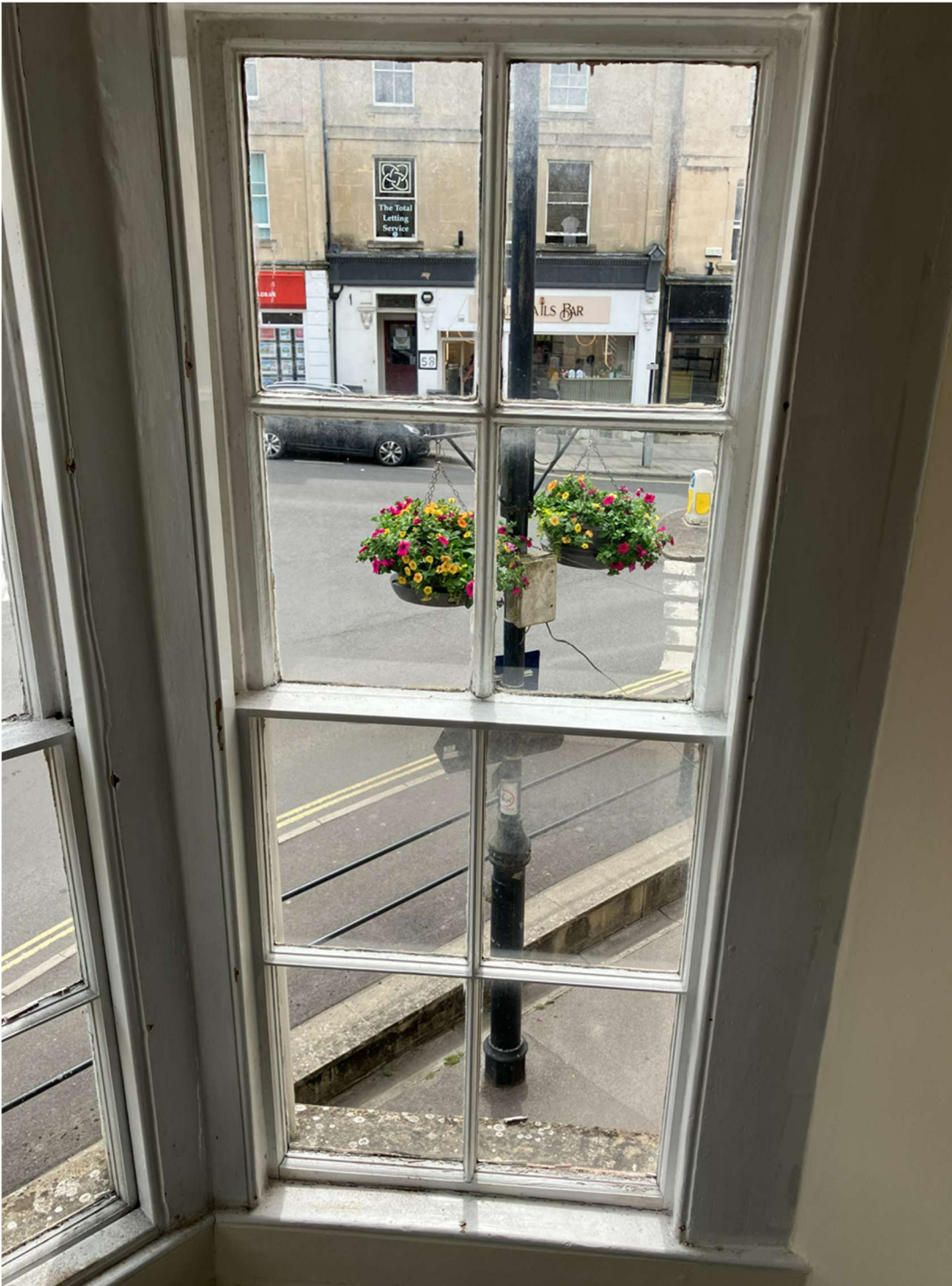
One example of a window with a possibly nineteenth century upper sash and a twentieth century replacement lower sash
