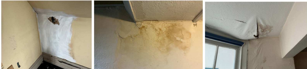
Roof leaks
