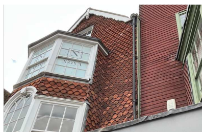
Front façade Club and Fishtail vertical hung tiles
