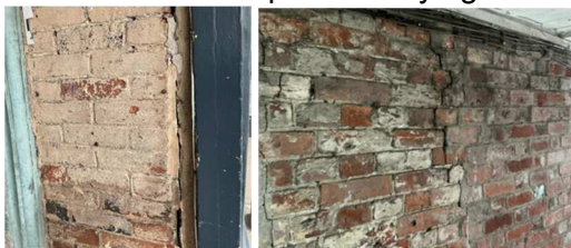
Minor work to wall on Chandler Yard – helifix repair
