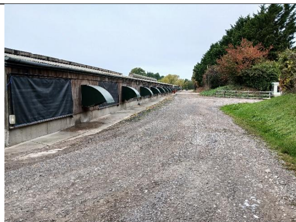
Plate 6. Hardstanding in the centre of the site.
