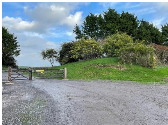
Plate 1. Access track comprising of hogging
