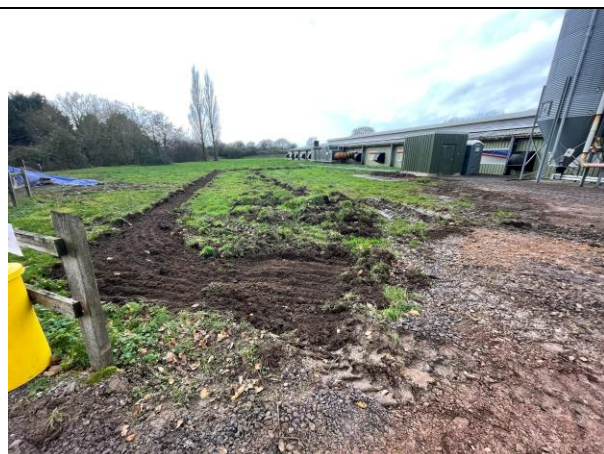
Plate 3. Soil Strip conducted under ECOW following CEMP guidance
