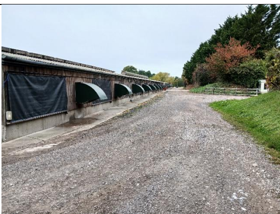
Plate 6. Hardstanding in the centre of the site
