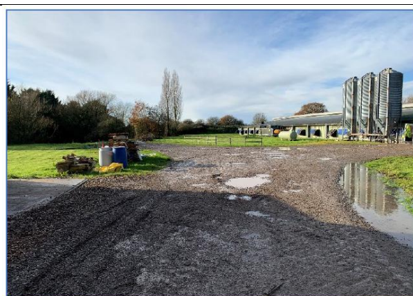
Plate 2. Access track comprising of hogging
