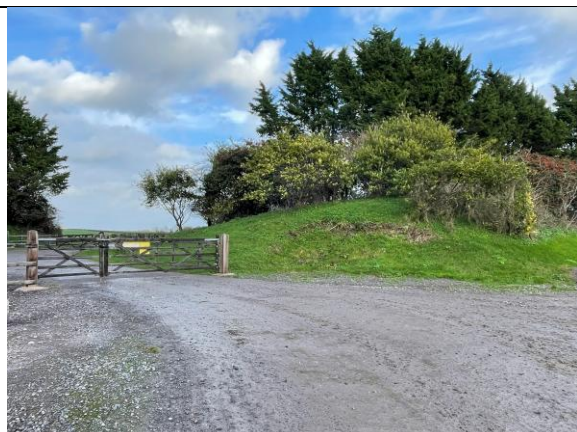
Plate 1. Access track comprising of hogging
