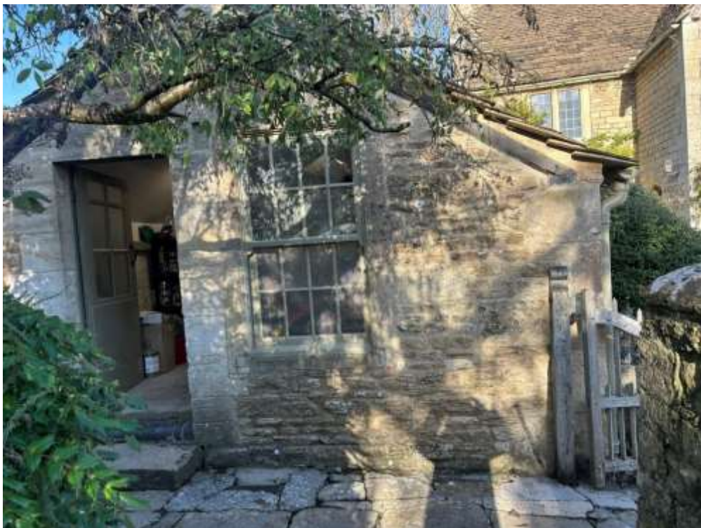
Workshop from the south, re-used sash window, concrete slab introduced to raise floor level can be clearly seen at the door threshold.
