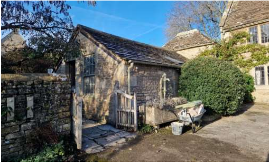
Workshop from the stable yard, re-used elements of dressed stone set within rubble masonry. Pavilion can be seen behind to the right.
