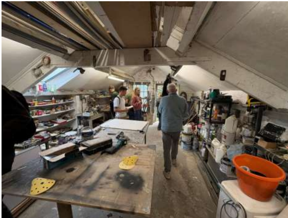
Workshop interior, modern construction, concrete floor slab to be removed to increase headroom.
