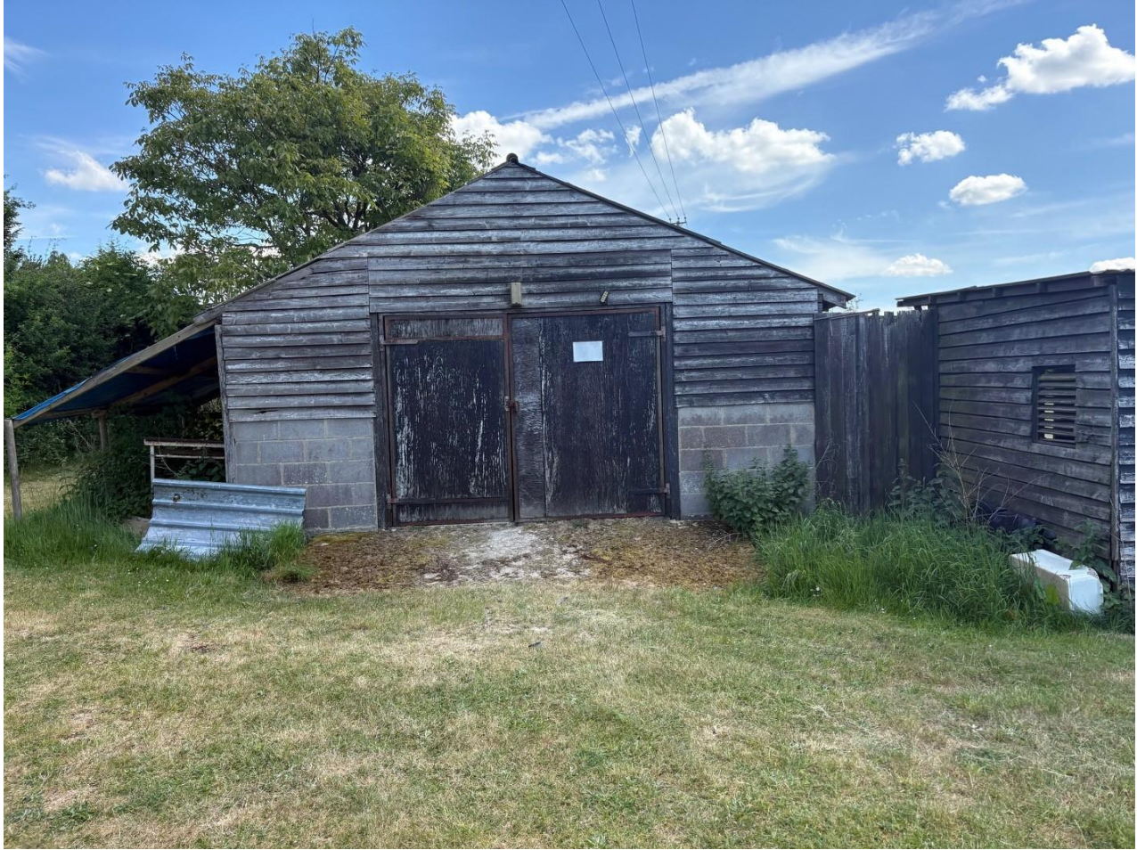
Photo 3 - Existing hardstanding at Building A. The proposed residential extension is predominantly located on existing hardstanding. The retained structure of Building A is visible behind.
