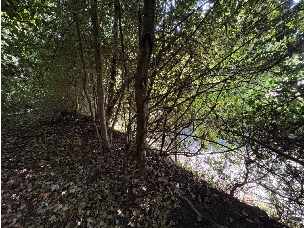
46-1043 Image 6 Holly, hawthorn and other vegetation above and adjacent to Upper Marsh Road encroaching on the highway.
