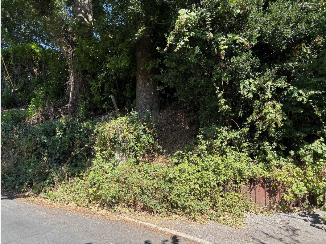
46-1043 Image 10 Pedestrian link from Damask Way with Upper Marsh Road with sheet piling on the edge of the footpath and adjacent to two mature oak trees.
