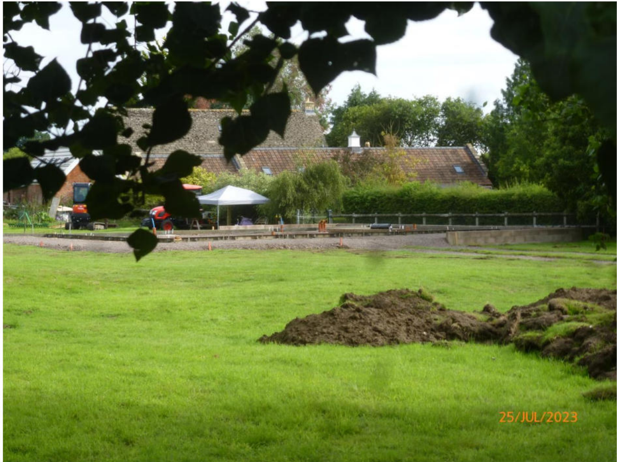
The picture above shows the new agricultural barn footings constructed in July 2023. The building visible behind are the stables building referred to as building no.2.
