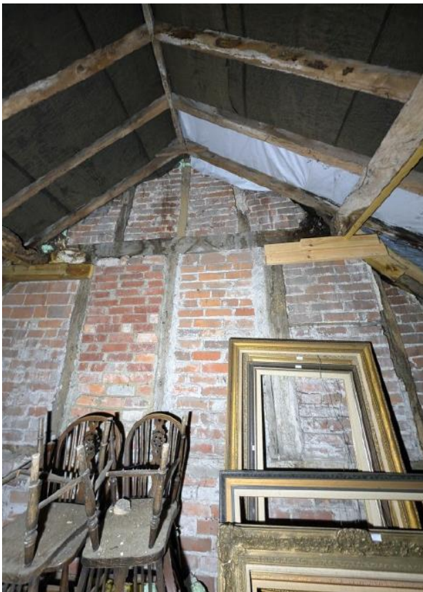
Fig.9 Timber-framing of The Old School House
