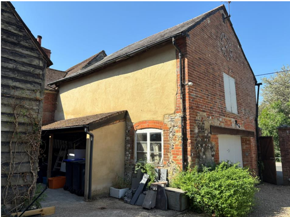
Fig.6 East side of the building; patch of stone and flint around a window
