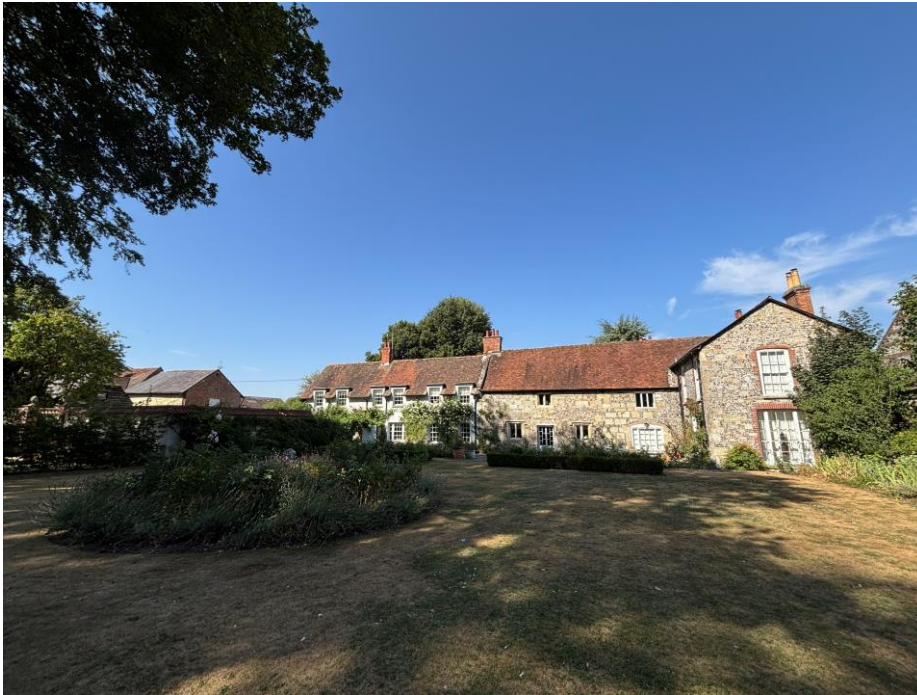
Fig.12 View from the garden looking towards the back of the house - outbuilding on the left
