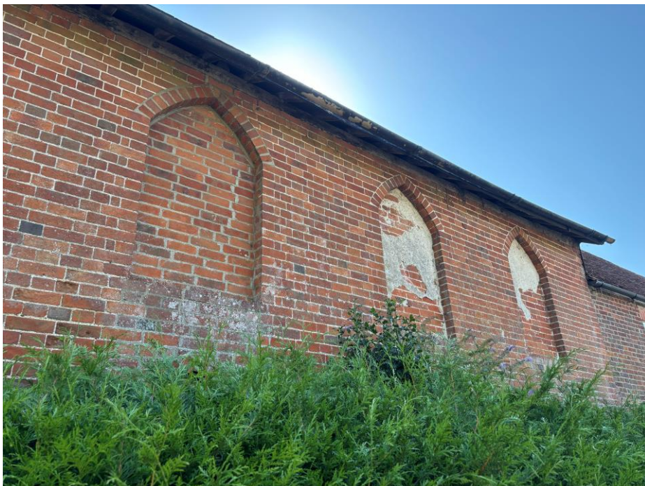
Fig.4 Blind Gothic-arched windows on the roadside elevation; remnants of a lime render finish on the two right-hand blind windows
