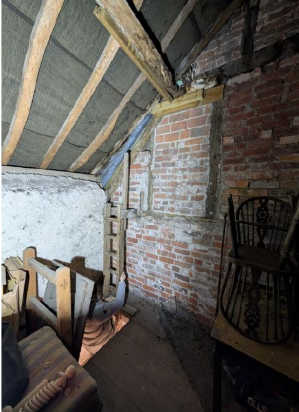
Fig.8 Loft hatch and ladder
