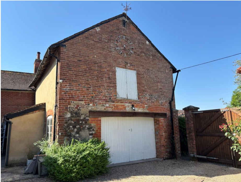
Fig.5 North gable of the outbuilding; modern opening with old stone and flint walling to the left
