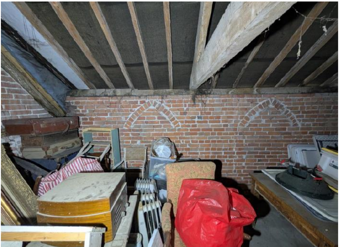
Fig.11 West wall – arches of the blind windows visible
