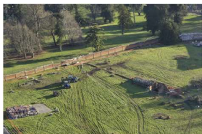
Spine Wall – Existing condition
