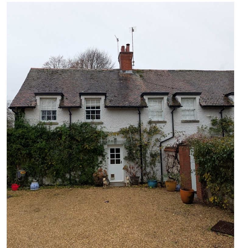
Existing Front Entrance
