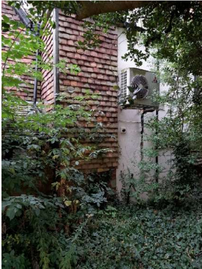
Fig. 4 Image of the north elevation
