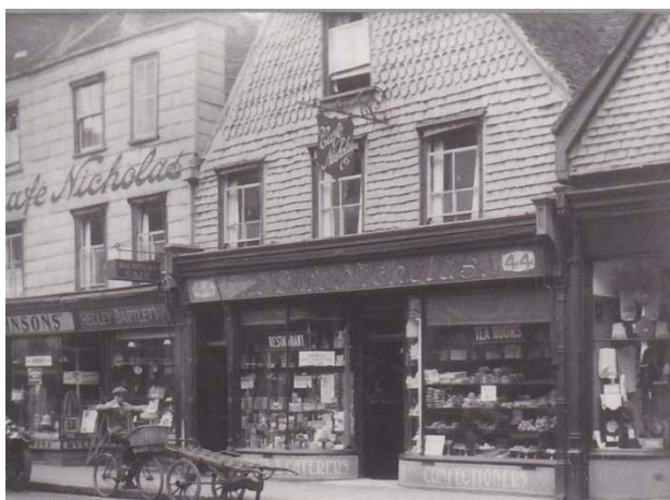
Fig. 10. 44 Silver Street in the 1920s still known as The Café Nicholas with a restaurant and tea rooms. The business extended into the first floor of 46 Silver Street. Note the tile hanging.
