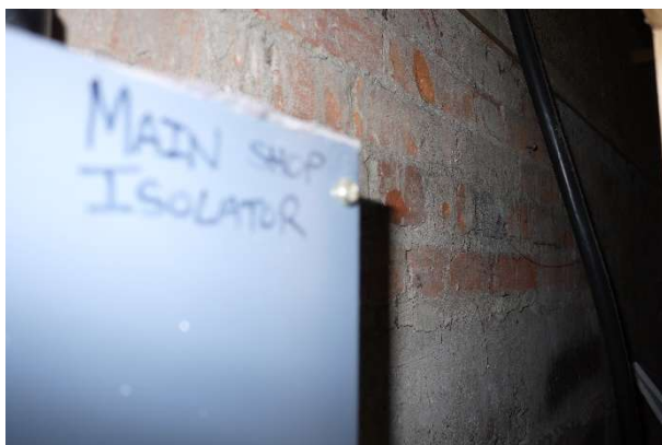
Fig. 6 Ground Image of the party wall between 44 and 42 glimpsed through a small opening at the back of the cupboard. Note the modern brickwork and sand/cement mortar joints
