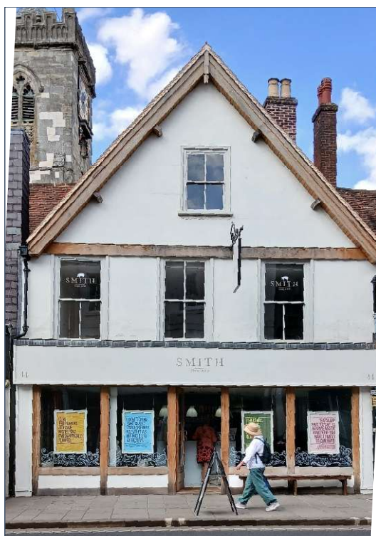
Fig. 1. View of the south side of the building.
