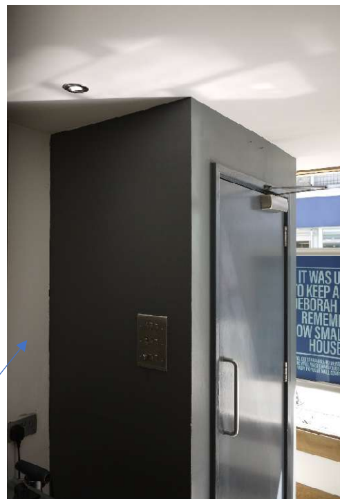
Fig. 7 Image of the service cupboard. The proposed door is to the left of the side wall of the cupboard
