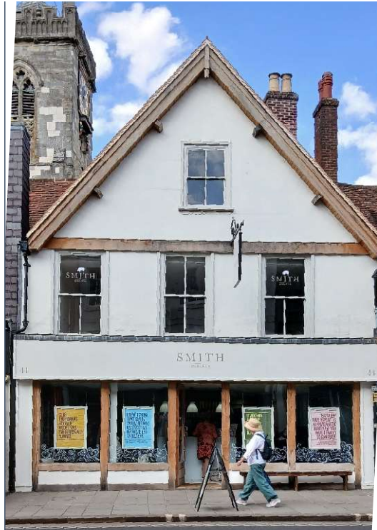
Fig. 1 Image of the main, south elevation
