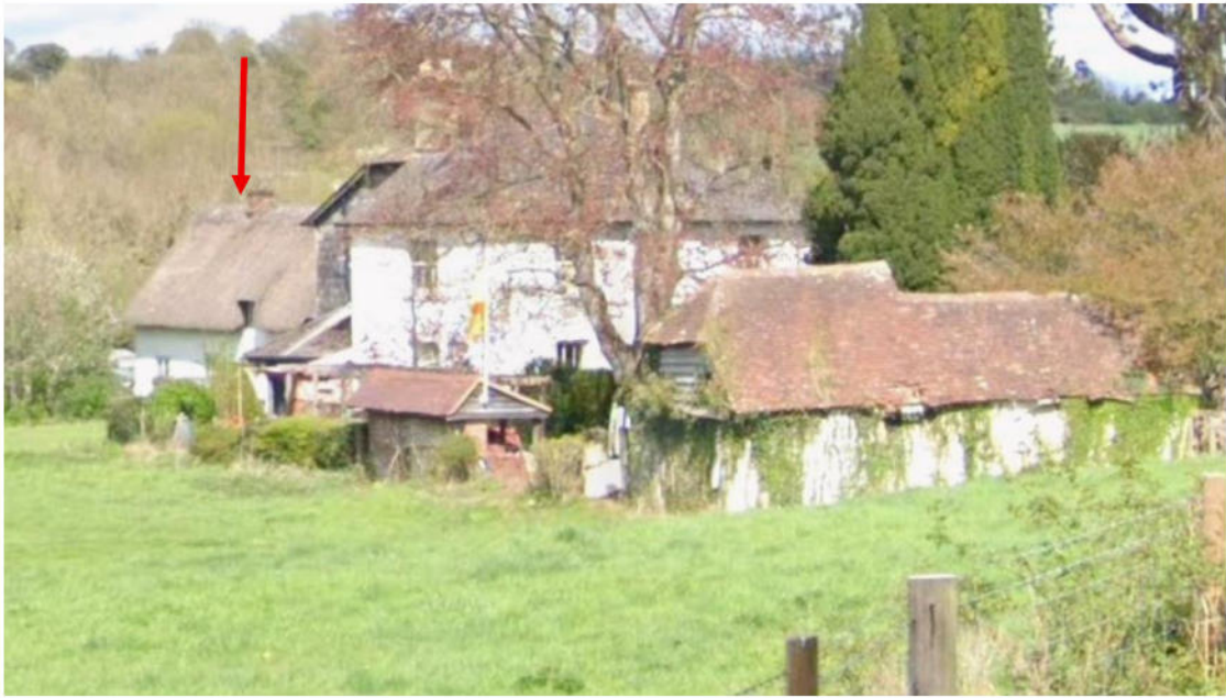
Fig.8 Close-up view from the south showing the juxtaposed building forms and variation in roof materials
